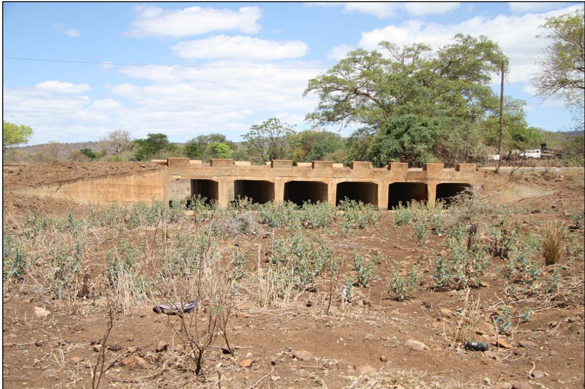
Figure 3. View of the existing culvert
