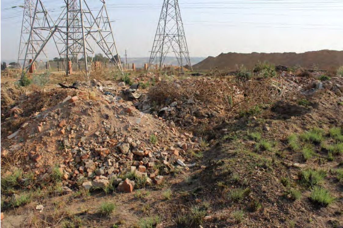
Figure 11: Site Characteristics (E)
