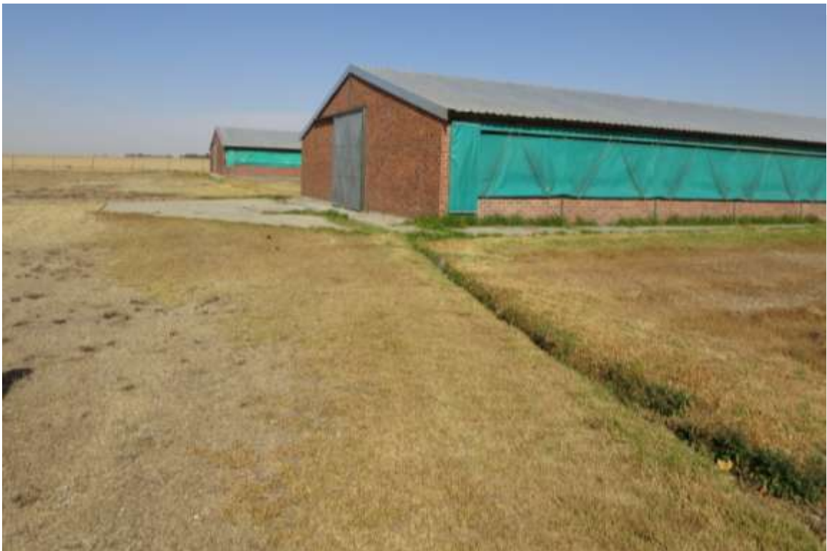
Figure 10: Photograph of an existing broiler house and wash water trench.
