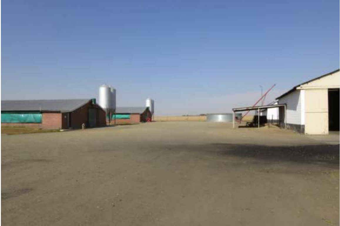
Figure 9: Photograph of the existing broiler houses in opposite direction to Figure 2.
