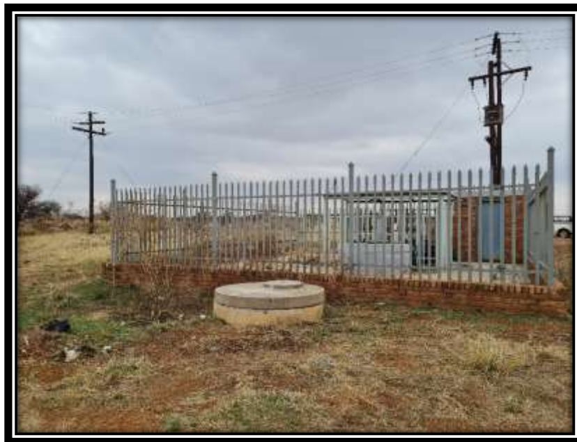
Photograph 8: Sewage pump station is located on the north-western corner.
