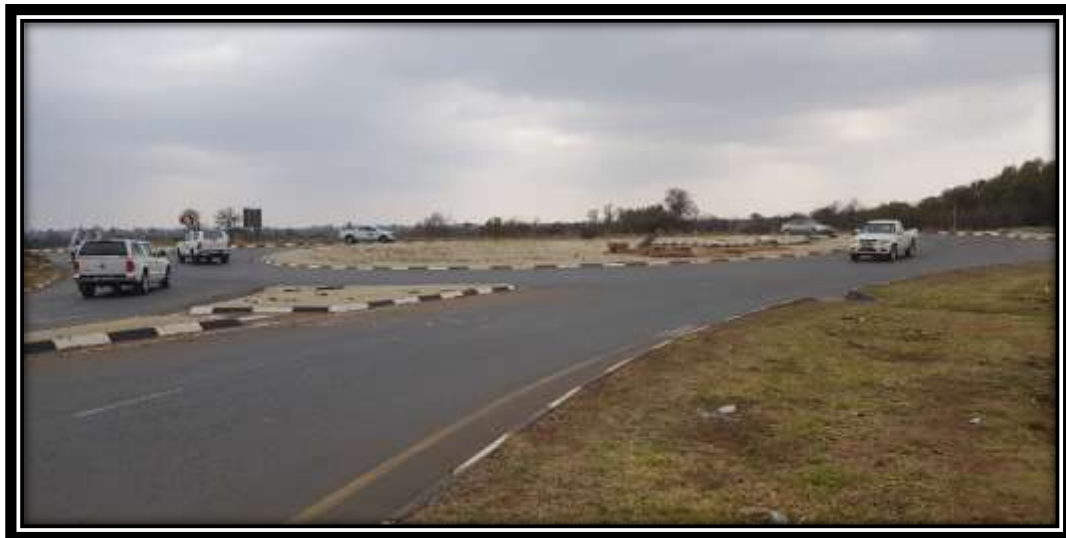
Photograph 2: The newly constructed traffic circle
