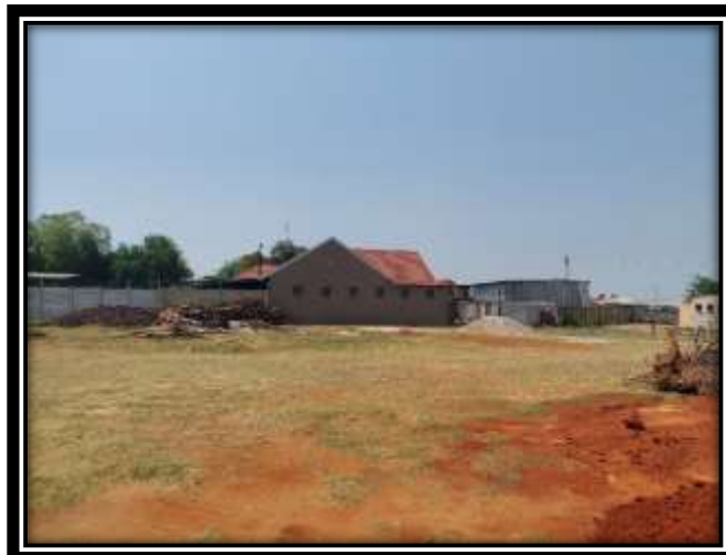
Photograph 3: Portion 3 is currently used for residential purposes. Illustration of the main house.
