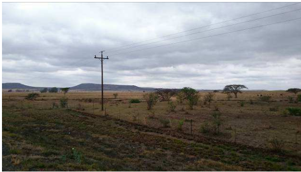
PLATE 13: Pipeline corridor within grazing lands. Area prone to erosion and dispersive soils.
