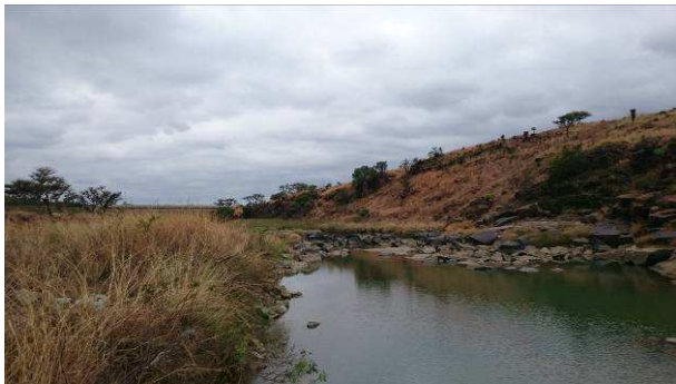
PLATE 23: Pipeline corridor the vicinity of the second Klip River crossing (upstream of the R103 crossing with sensitive riparian vegetation area in the foreground).
