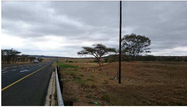
PLATE 11: Pipeline corridor in the vicinity of the D142 intersection.
