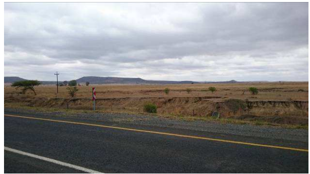
PLATE 124: Pipeline corridor within grazing lands. Gully erosion evident in the foreground.
