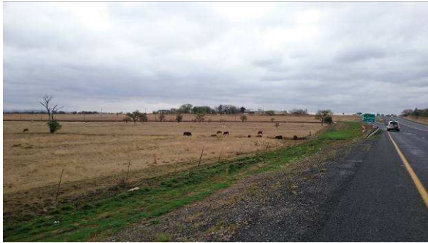
PLATE 19: Pipeline corridor approach to the R103 offramp (grazing lands).
