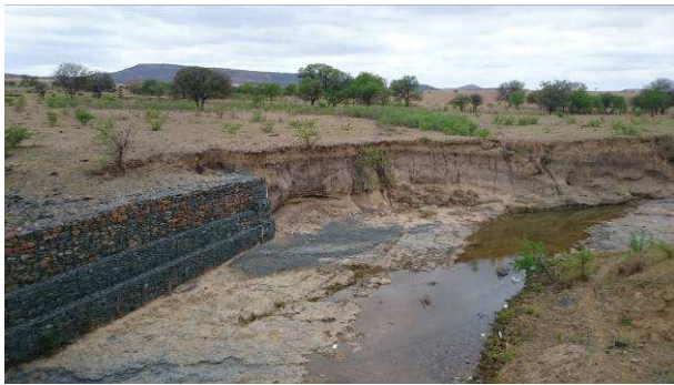
PLATE 15: Pipeline corridor, upstream crossing of the Flagstone river. Area prone to erosion and dispersive soils.
