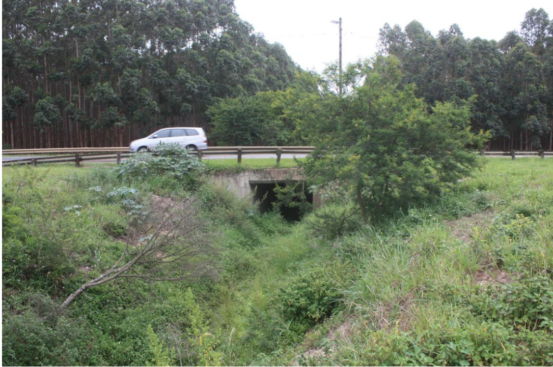
Fig. 9. Image of wetland system 2 near road culvert.
