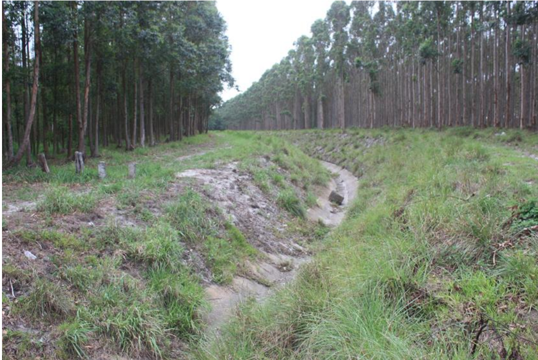
Fig.7. Sluice drain on Wetland 1.
