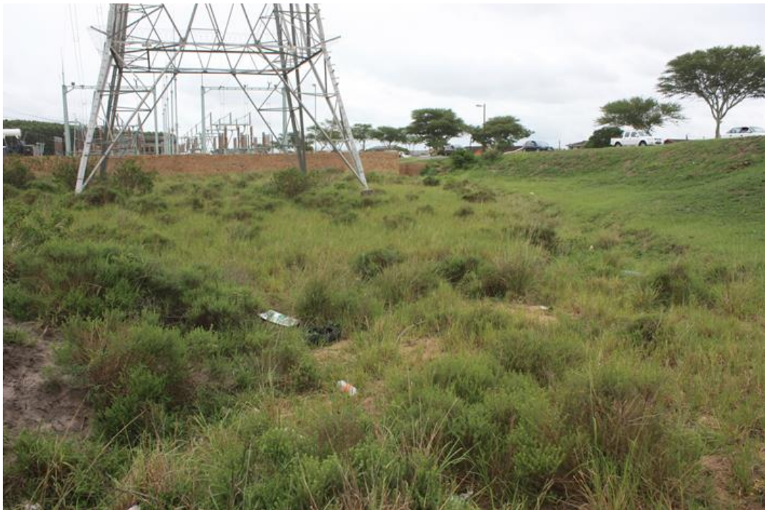
Fig. 10. Image of wetland system 4, with substation in background.
