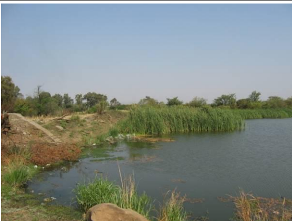
Photo 17 (Dam Wall South)
