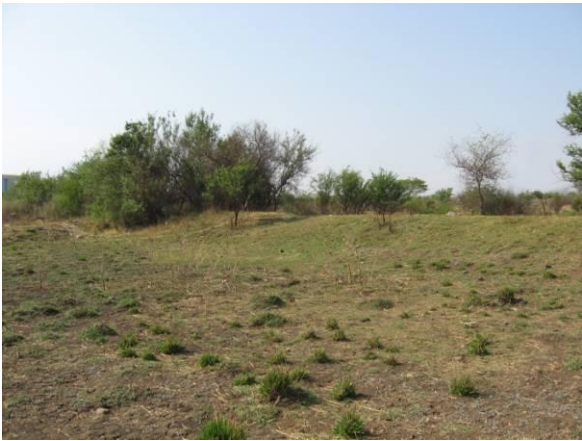
Photo 13 (Dam Wall North)
