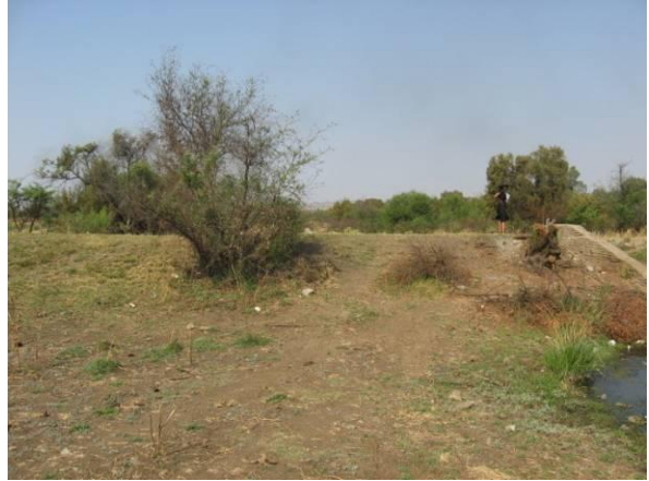
Photo 14 (Dam Wall North)
