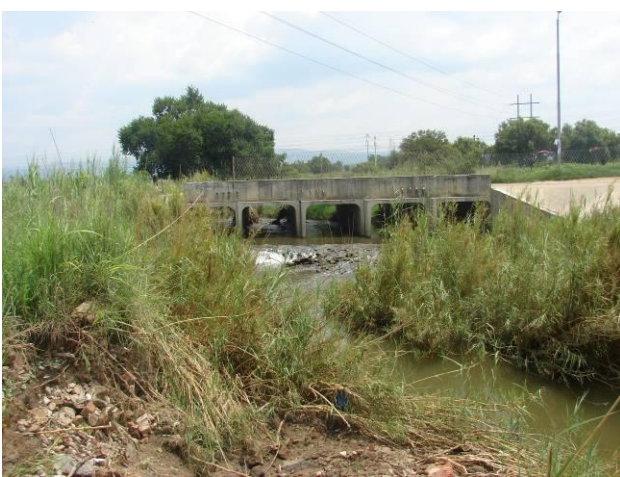
Photo 32 Phala road crossing culvert
