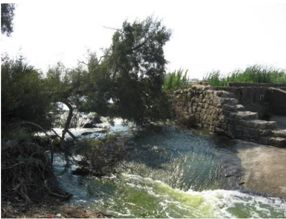
Photo 27 (The spillway itself)
