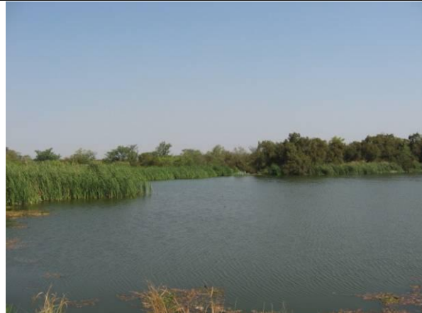
Photo 18 (Dam Wall South)
