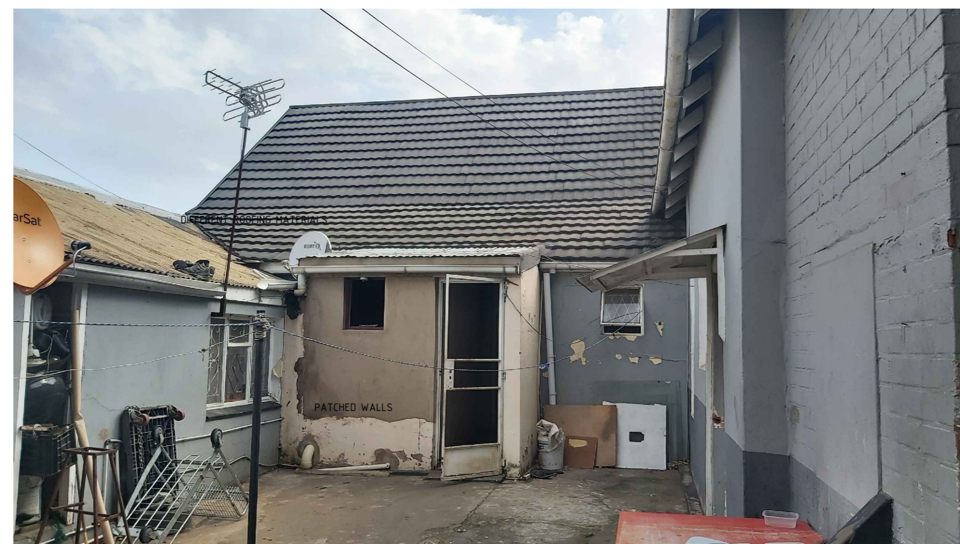
REAR OF THE BUILDING
