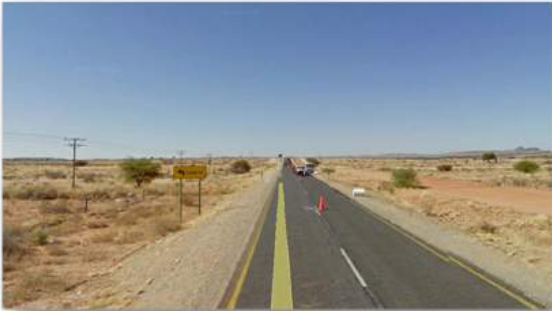
Photo 1.1: R27 towards the south (taken towards Kenhardt). The board shows “Loop 14”, located to the left, which is accessed via the Transnet Service Road. (Image source: Google, 2010)
