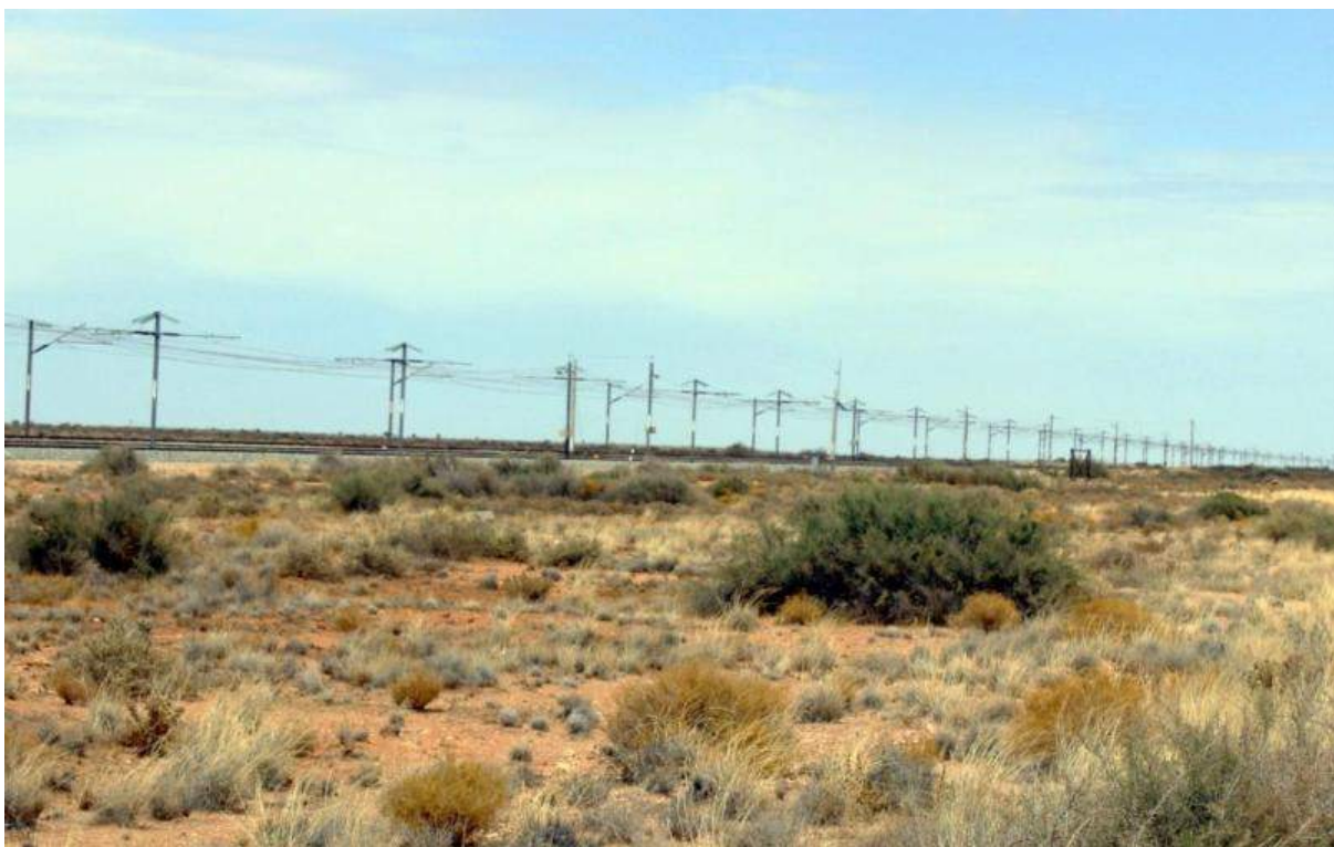
Figure 5: Photograph depicting Saldanha-Sishen iron ore railway bordering the south-eastern side of the project area (CSIR, 2016a; photo credit: Henry Holland).
