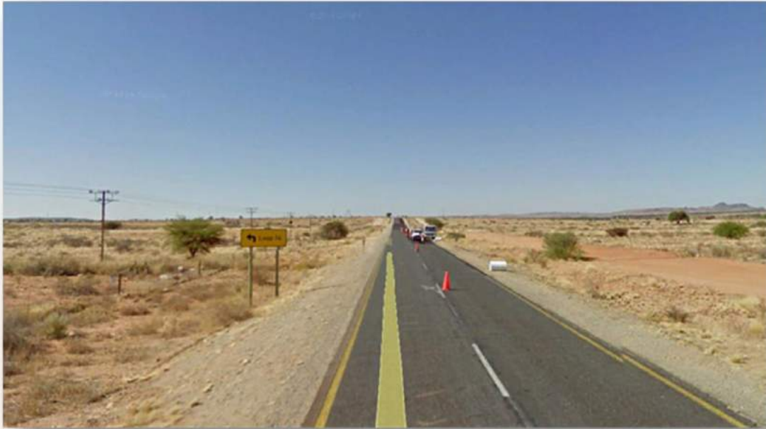
Photo 1.1: R27 towards the south (taken towards Kenhardt). The board shows “Loop 14”, located to the left, which is accessed via the Transnet Service Road. (Image source: Google, 2010)
