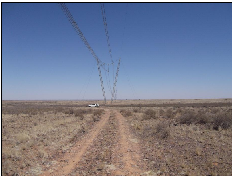
Figure 5-3: Existing two track service road below 400 kV CRS transmission line
