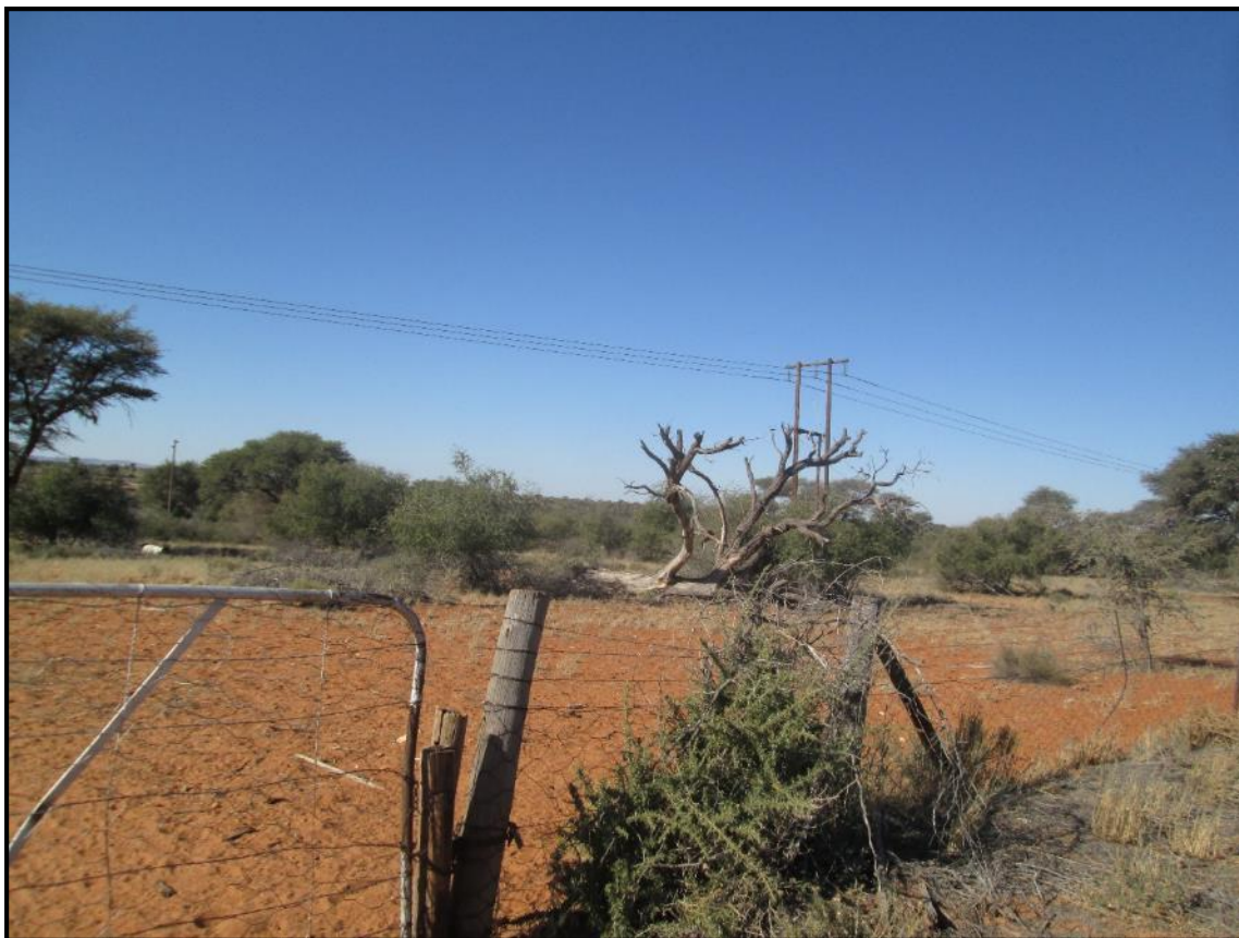
Plate 5: View of the Powerlines Along the R308 Road to the West of the Proposed Site and of an Entrance to One of the Farm Houses.
