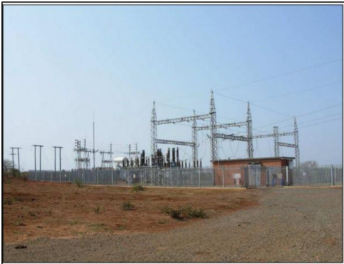
Plate 1: Example of a typical substation structure
