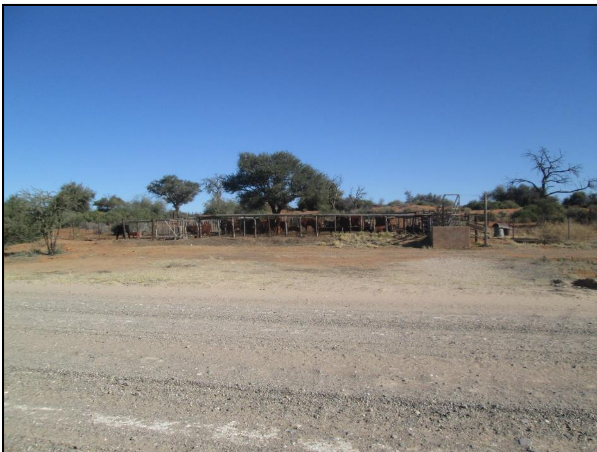
Plate 4: View of the Cattle Kraal to the West of the Substation.
