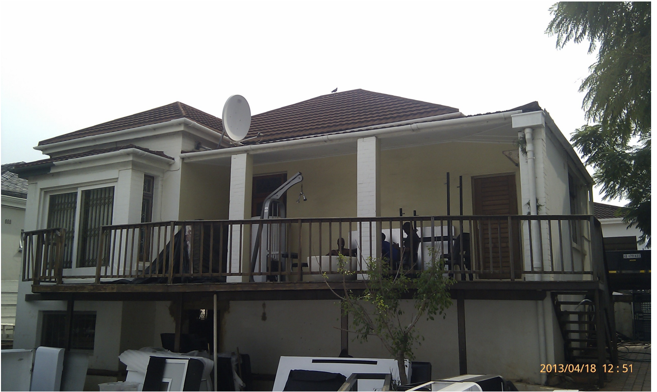
Main House / South East Elevation / deviation A
