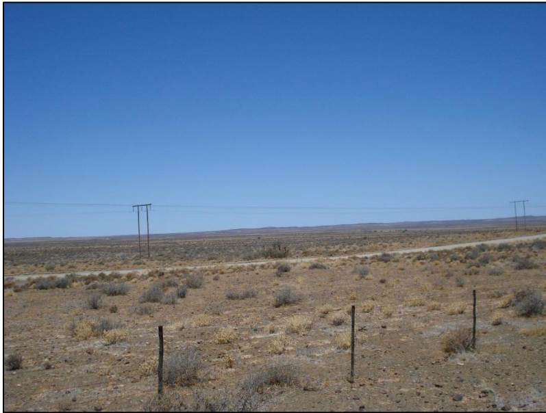
Figure 5-2: Existing transmission line that runs along the gravel road at the Loeriesfontein site
