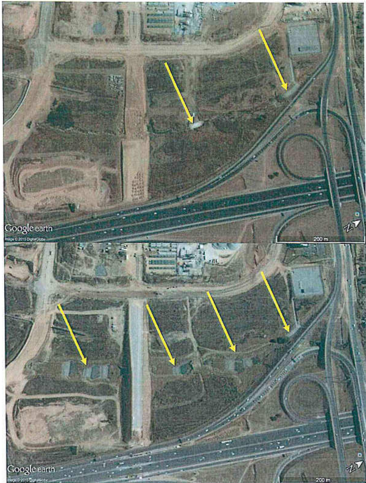
Figure 27 Google Earth images from 2014/08/10 (top) and 2015/06/10 (bottom) indicating rehabilitation and stabilisation work within the watercourse
