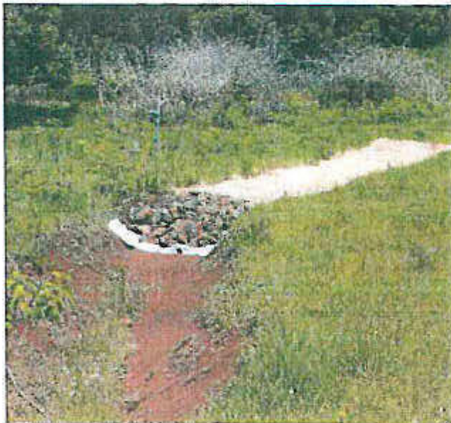
Figure 4: Filling and mulching of gullies
