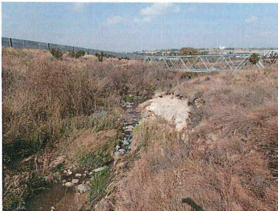
Figure 2 Eroded channel of the watercourse indicating extensive cutting into the original wetland soils
