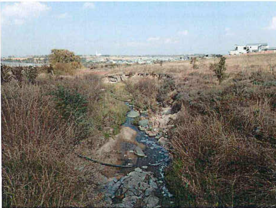
Figure 3 Eroded channel of the watercourse indicating extensive cutting into the original wetland soils.
