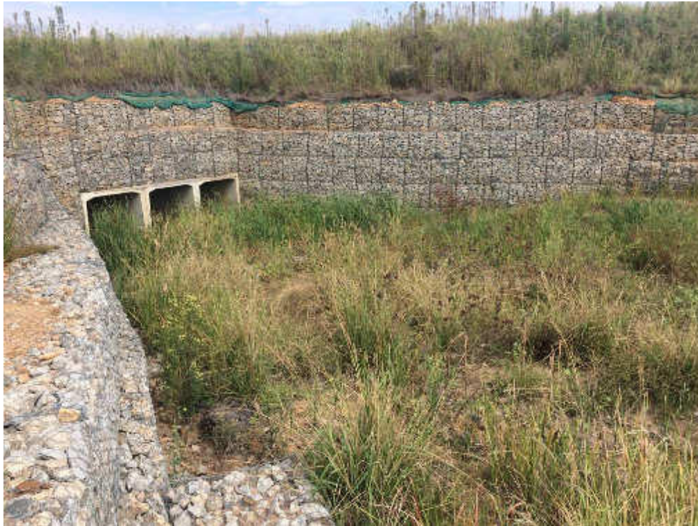
Figure 3 Gabion and culverts used to rehabilitate the drainage line.
