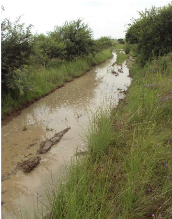
Figure 11: View of a section of flooded road in the southern section of the project footprint
