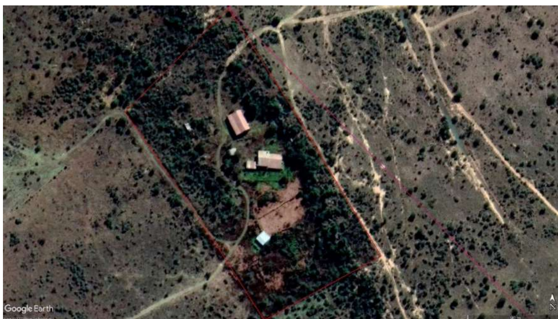
Figure 24: View of site Os1-03, showing the extent and the number of buildings (Google Earth satellite imagery)
