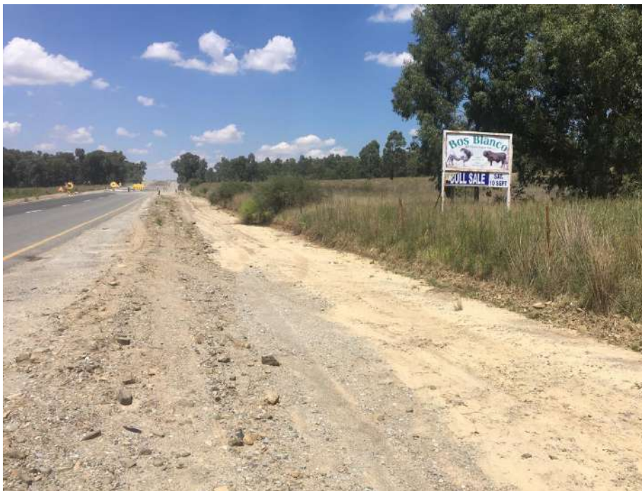
Figure 3-8: Construction on R76
