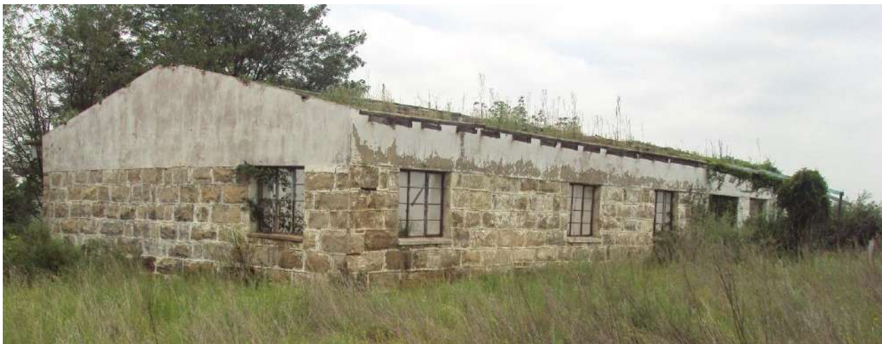
Figure 25: View of the rear elevation of the main farmhouse, showing the sandstone construction material
