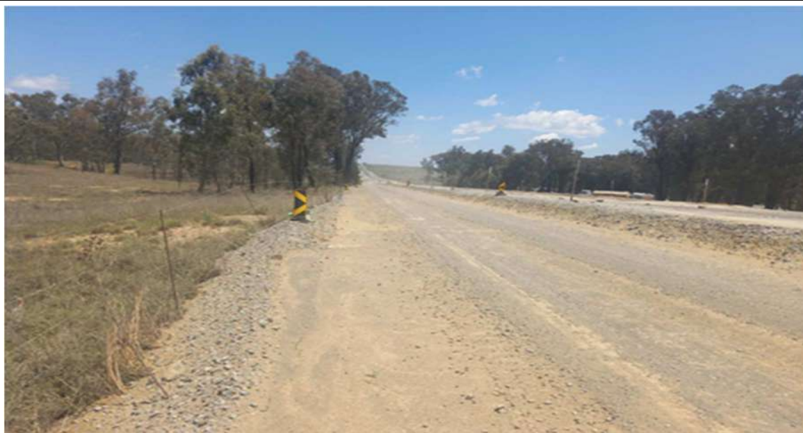
Roadworks along the R76
