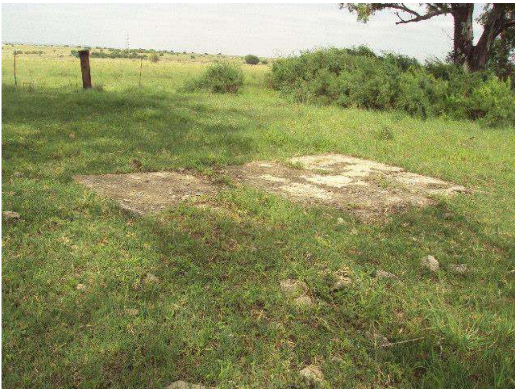
Figure 18: View of concrete foundation in the area of Os1-01)
