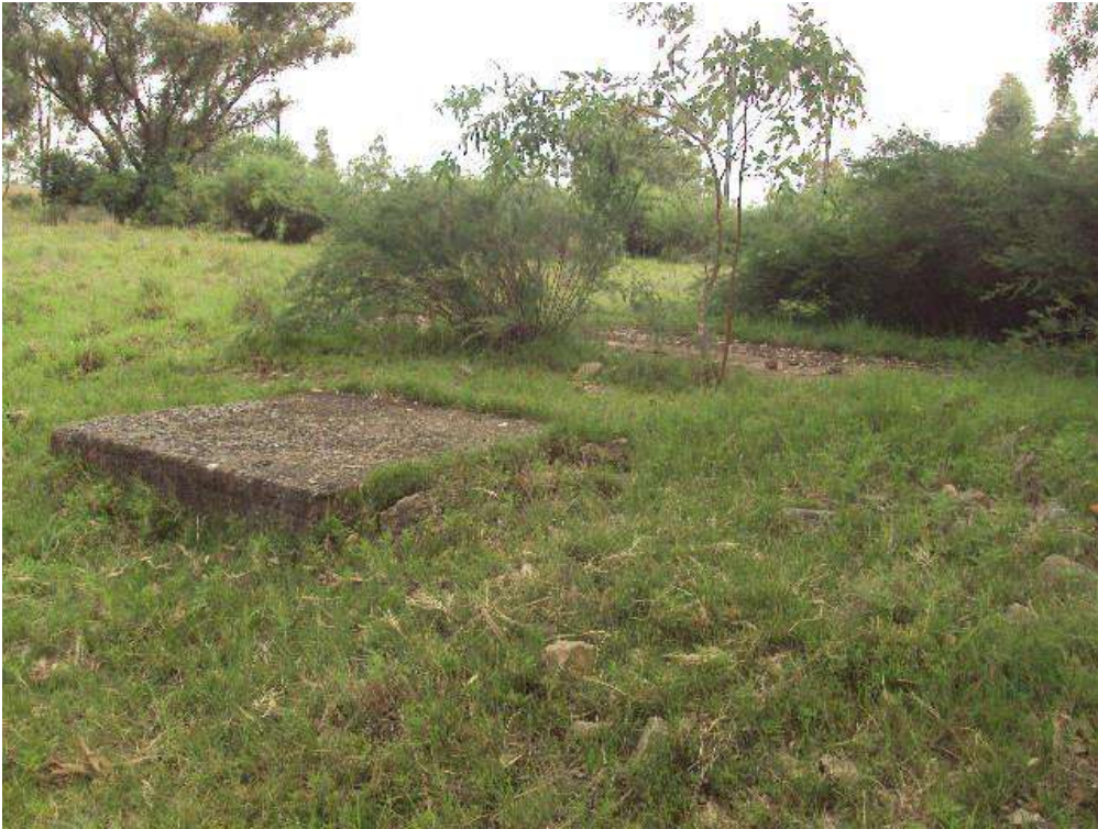
Figure 19: View of concrete foundations of multi-roomed building at Os1-01B
