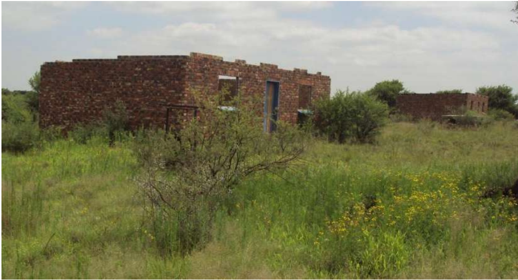
Figure 22: View of the two house structures at Os1-02. Note the dense surrounding vegetation
