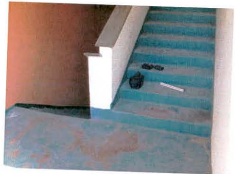
Internal stair from first to second floor. Four of these stairs are to be demolished. Refer to floor plans.
