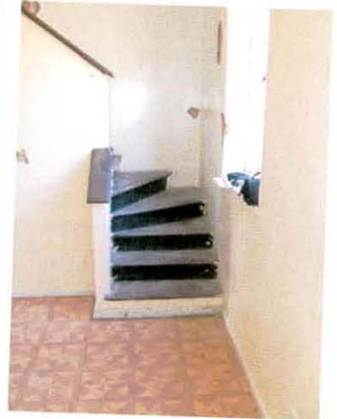
Internal stair from first to second floor. Four of these stairs are to be demolished. Refer to floor plans.
