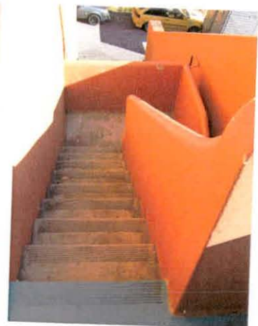
External escape stair.
