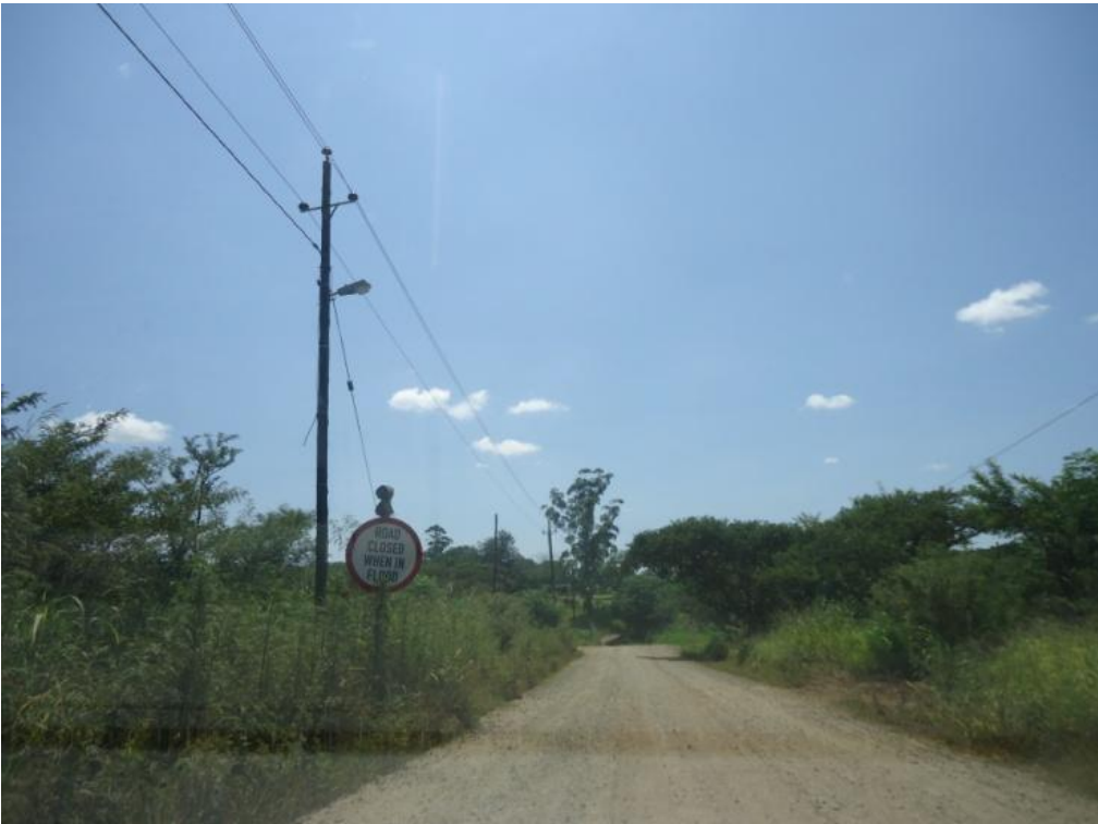
Grimthorpe avenue gravel section to be upgraded.
