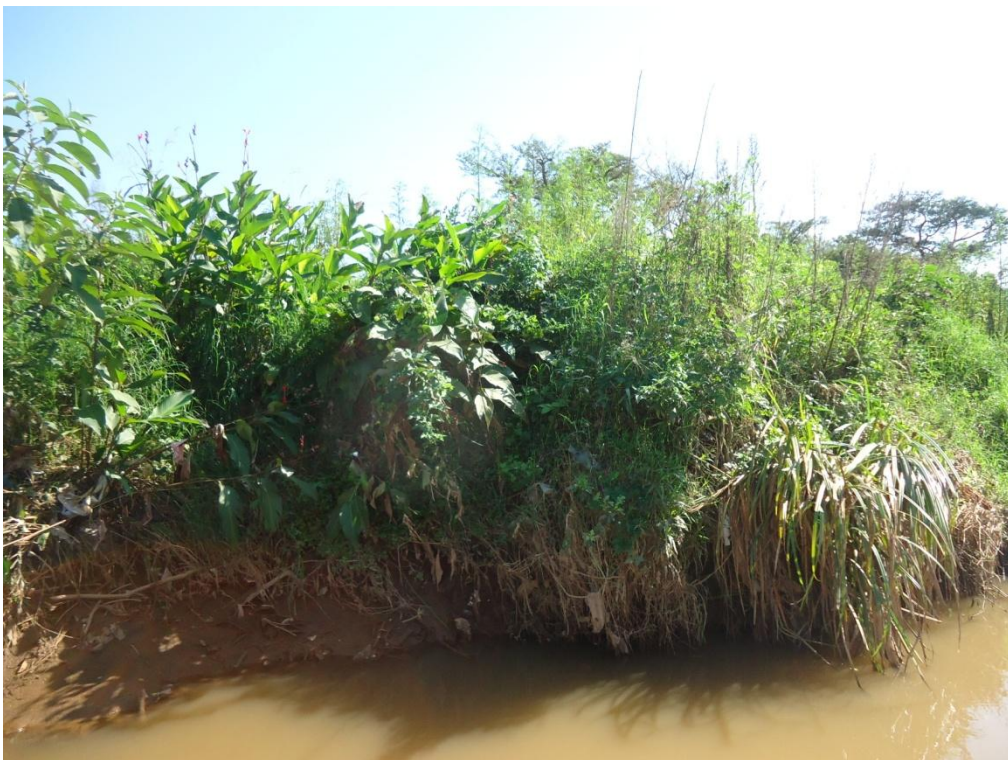
Image of weeds and scour at the immediate upstream bank.
