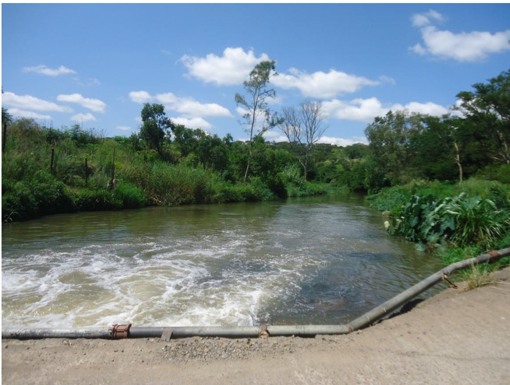
Downstream side of existing bridge.
