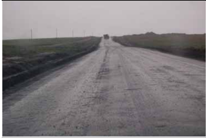
Figure 8.6 Dust Mitigation (Chemical Surface Treatment) on Public Roads to Panbult Siding
