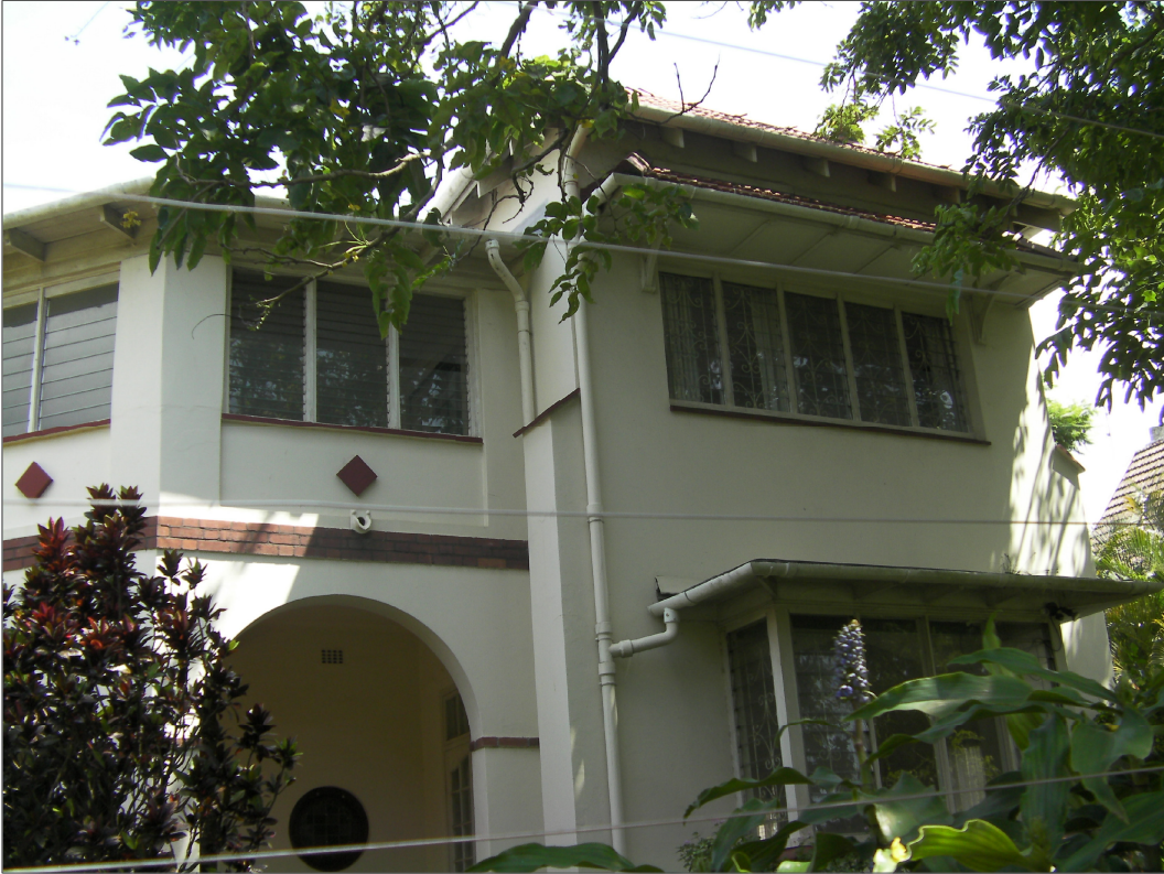
PHOTOGRAPH 1 ---- FACADE OF EXISTING BUILDING
