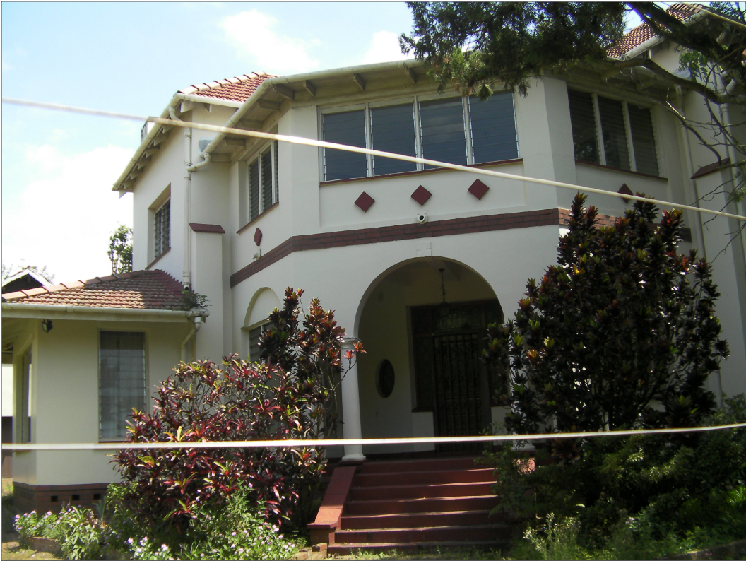
PHOTOGRAPH 2 ---- FACADE OF EXISTING BUILDING
