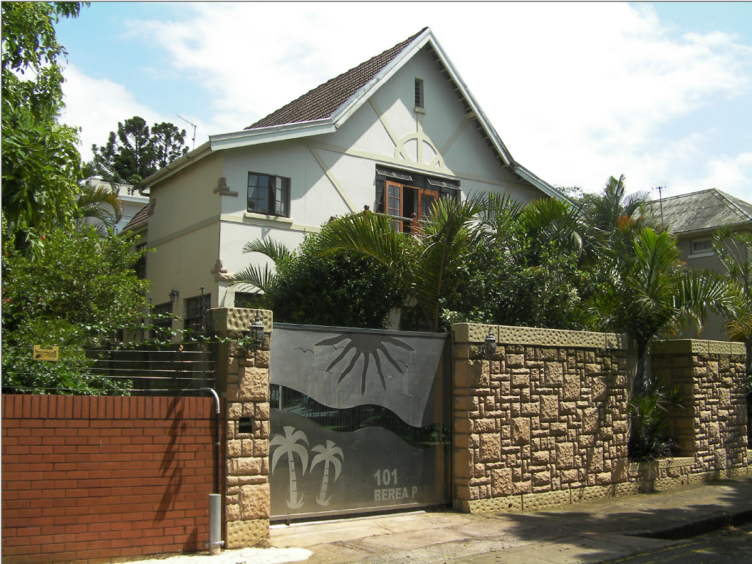
PHOTOGRAPH 6 ----- FACADE OF ADJACENT NEIGHBOURS BUILDING
