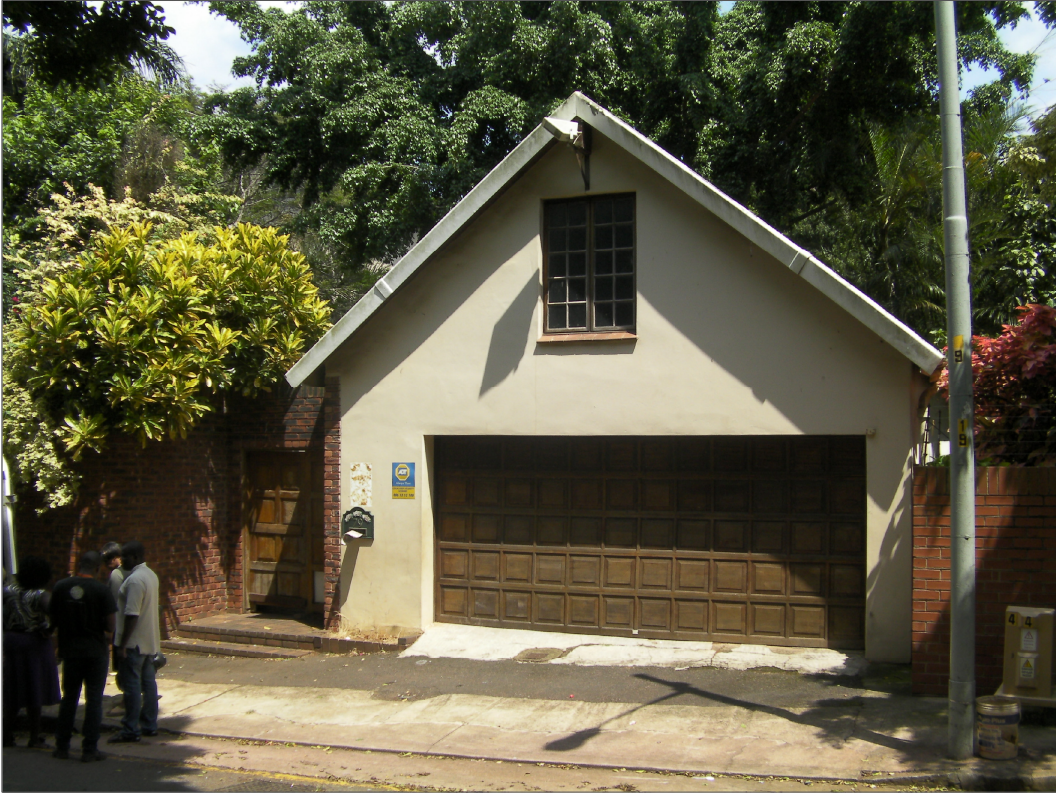
PHOTOGRAPH 7 ----- FACADE OF ADJACENT NEIGHBOURS BUILDING
