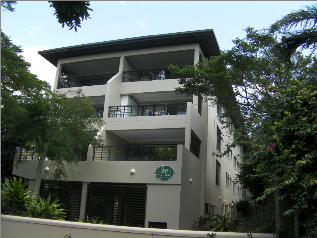
PHOTOGRAPH 8 ----- FACADE OF NEW DEVELOPMENT COMPLETED RECENTLY - TWO SITES AWAY
