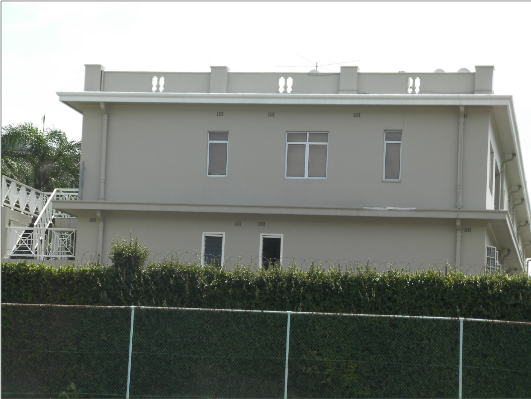
PHOTOGRAPH 10 ----- FACADE OF EXISTING NEIGHBOURING BUILDING AT THE REAR (RIGHT HAND SIDE)
