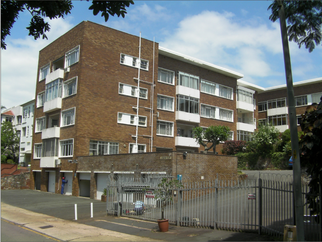
PHOTOGRAPH 9 ----- FACADE OF ADJACENT BUILDING - 3 SITES AWAY
