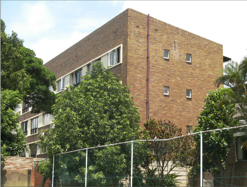
PHOTOGRAPH 11 ----- FACADE OF EXISTING NEIGHBOURING BUILDING AT THE REAR (LEFT HAND SIDE)
