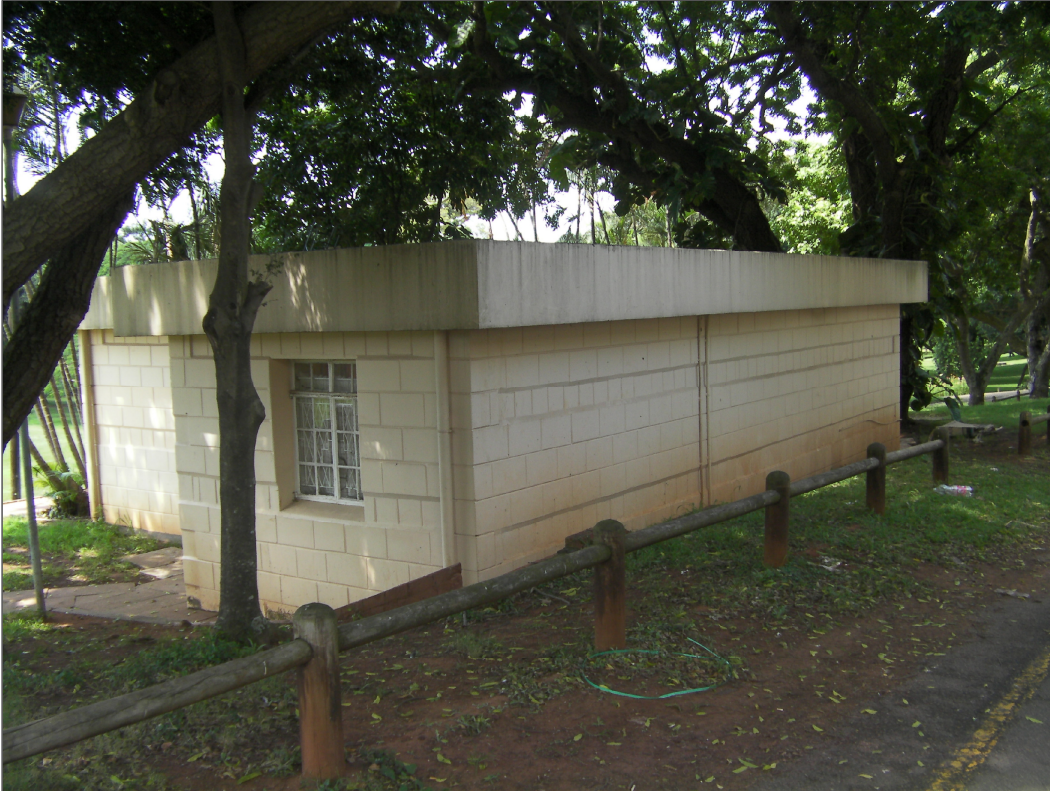
PHOTOGRAPH 13 ---- FACADE OF OPPOSITE CHANGEROOM OFFICE TO MUNICIPAL SOCCER FIELD (NEW BLOCK)
