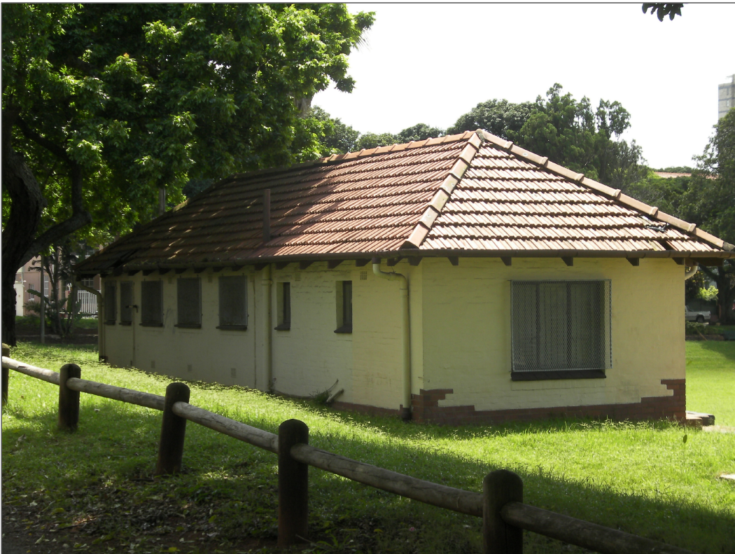
PHOTOGRAPH 14 ---- FACADE OF OPPOSITE CHANGEROOM OFFICE TO MUNICIPAL SOCCER FIELD (OLD BLOCK)
