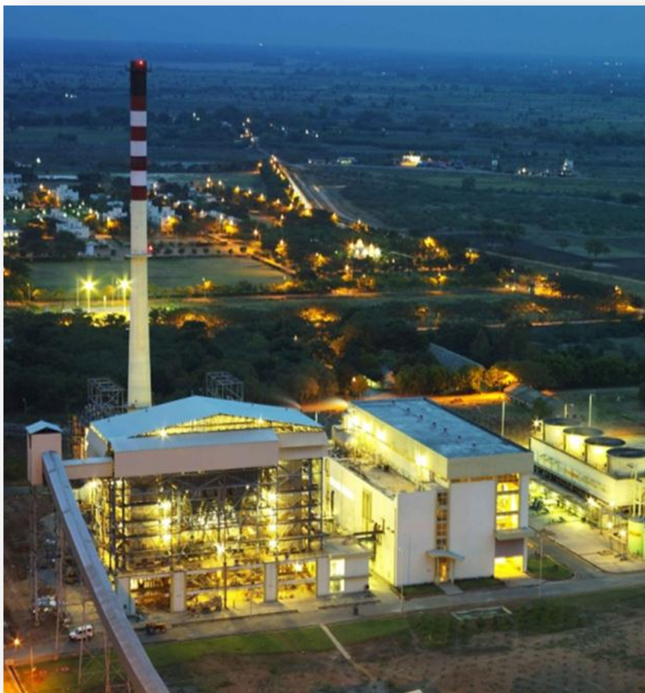
Figure 3-3: Representation of similar power station
