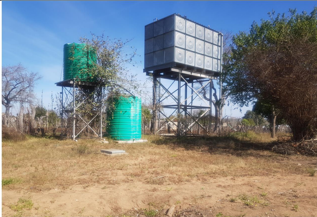
Elevated 0.079 Ml steel tank, Seville
