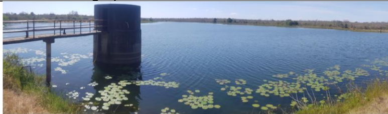
Thorndale Dam and pumping station
