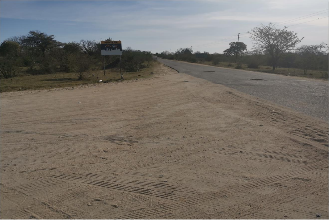
Figure 7 Access Road – internal street
