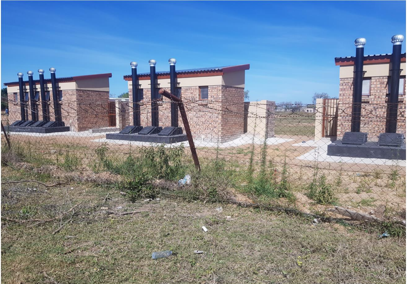
Figure 15 Enviro-Loo existing toilets at Seville school
