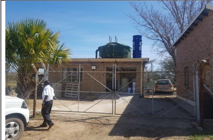
Thorndale Dam WTW
