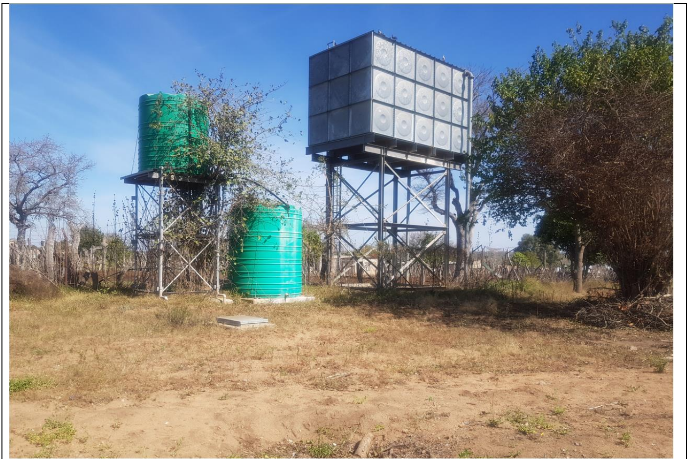
Elevated 0.079 Ml steel tank, Seville
