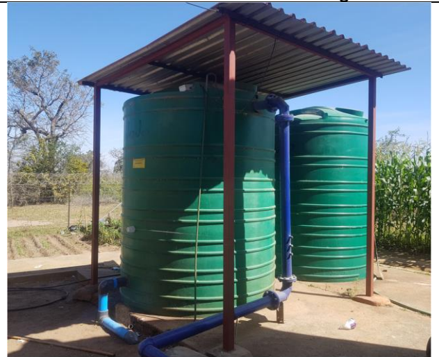
Potable water storage tank. One connected and one yet to be connected
