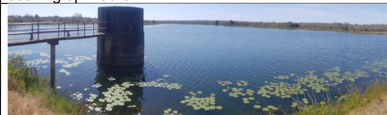
Thorn Dam and pumping station Thorn Dam, Seville, Bushbuckridge
