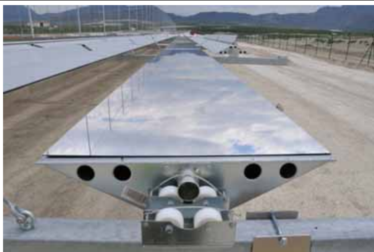
Figure 2.2: Primary reflector (Source: Novatec)
