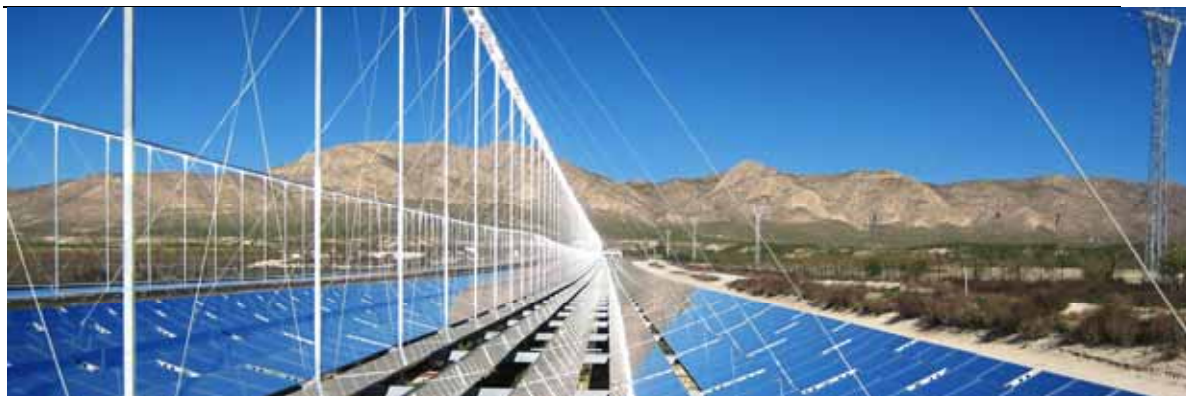
Figure 2.1: Linear Fresnel technology (Source: Novatec)
