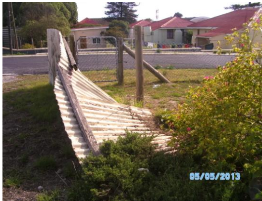
Part of fence laying down
