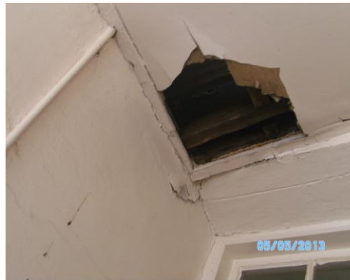
Condition of the ceiling
