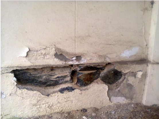
Condition of plinth
