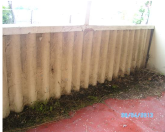
Condition of the porch
