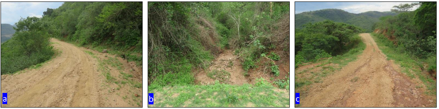
Figure 12: (a): Steep gradient where the pipeline follows the existing road at WC16; (b): Numerous watercourses were noted to have large amounts of loose sediment (WC18); (c): Pipeline predominately crosses the watercourses along existing roads (WC20).
