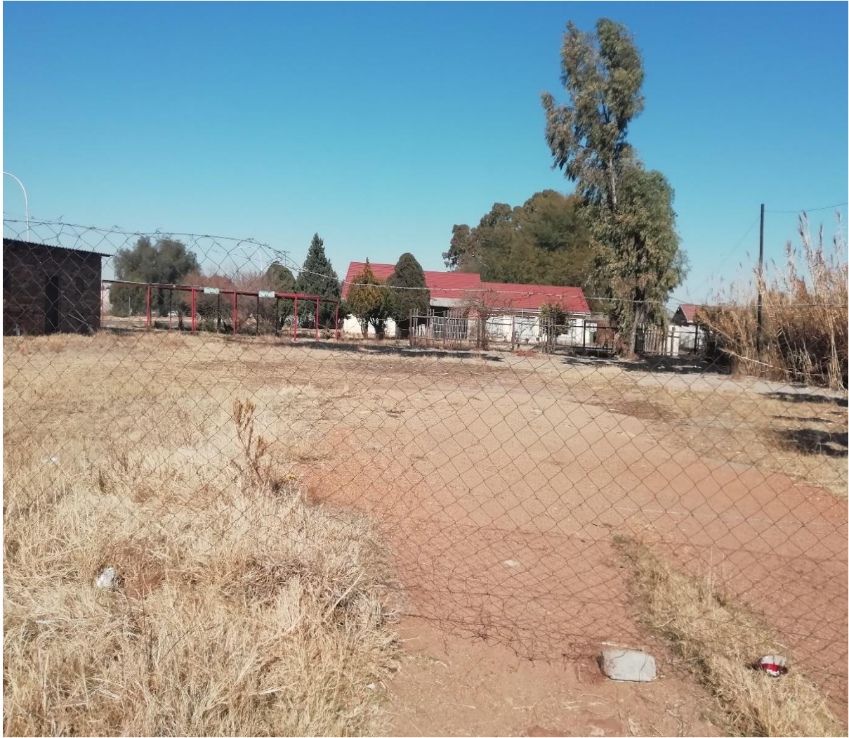
1.4 site camp after the contractor left the site
