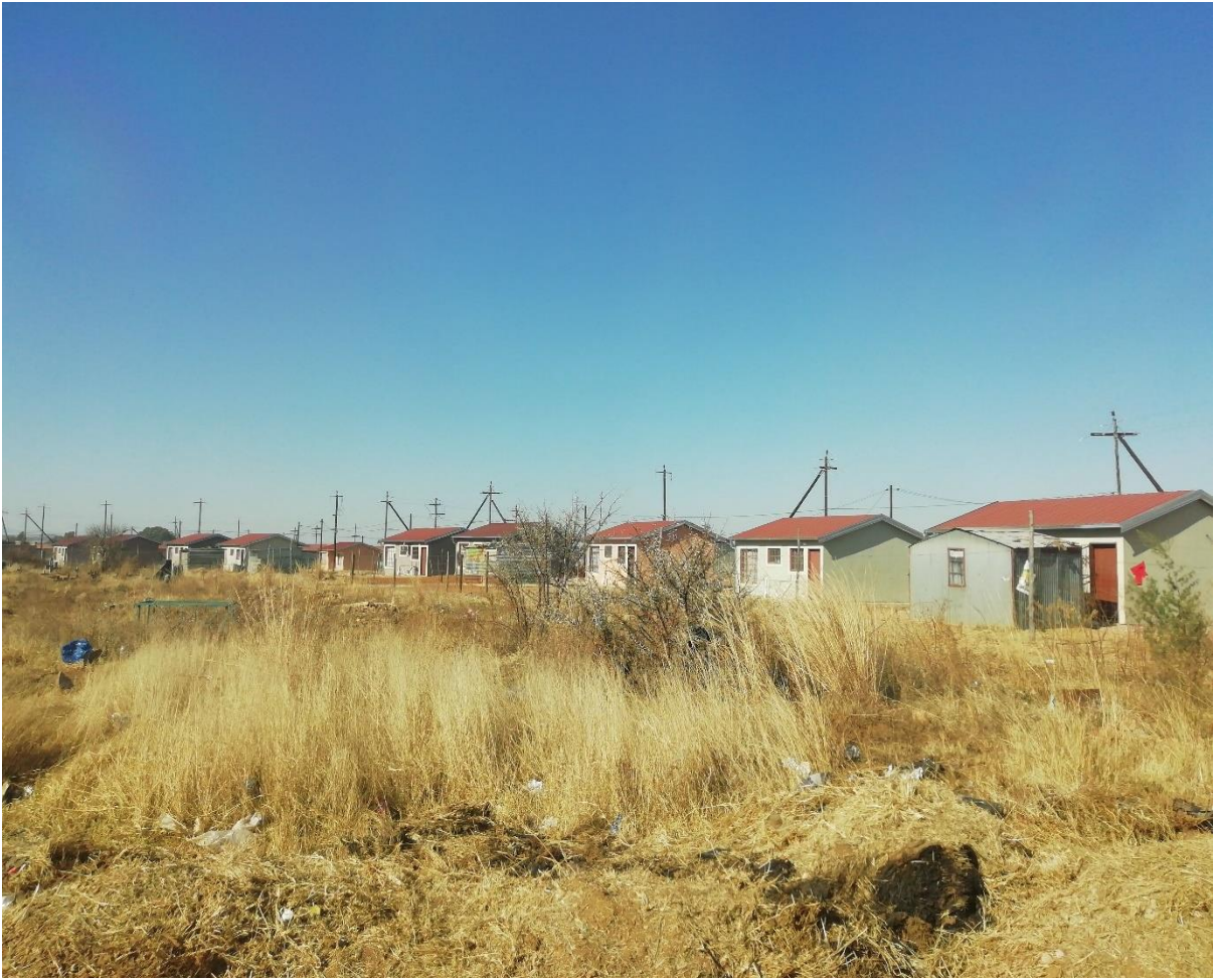
3.1 constructed electrification line
