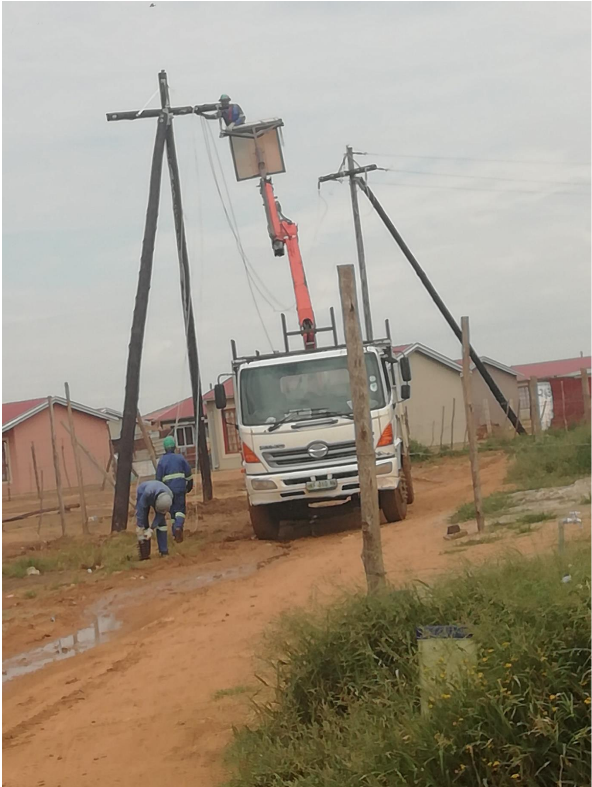
3.4 truck stringing the line under construction
