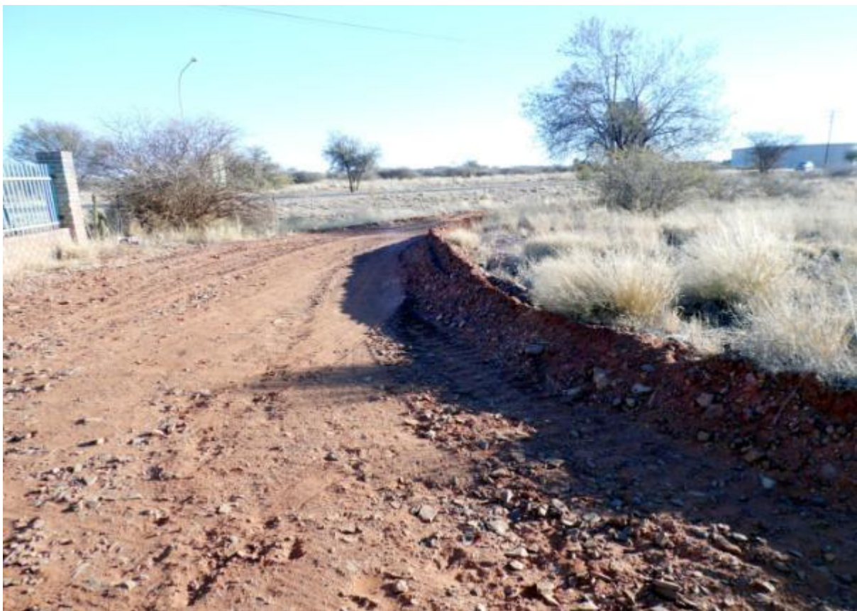
Figure 14: Road cut into the deposit of Townlands on the north side of Frikkie Meyer Street behind the Equestrian Club fence.
