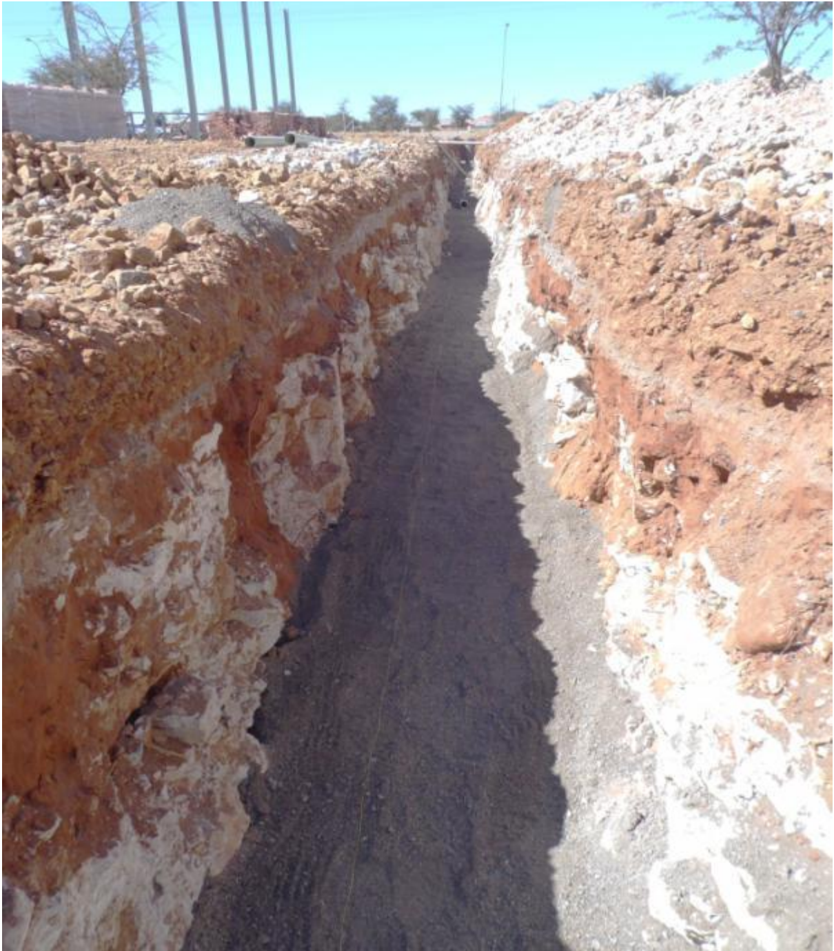
Figure 37: Developer trench from the centre of the trench looking east (deposit is mostly calcrete with some sand)
