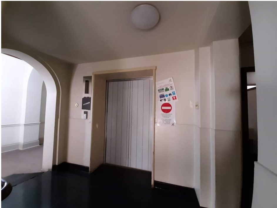
Fig. 60_Goods Delivery Lift replaced on second floor level (Source: tsica heritage consultants, 09.07.2019)
