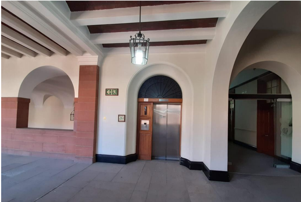
Fig. 57_Passenger Lift replaced on second floor level (Source: tsica heritage consultants, 09.07.2019)
