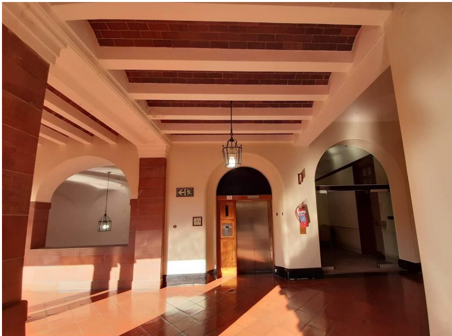
Fig. 54_Passenger Lift replaced on second floor level (Source: tsica heritage consultants, 09.07.2019)
