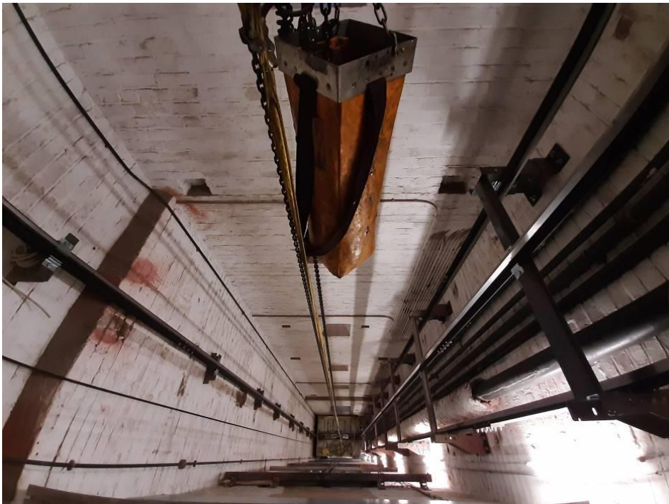
Fig. 85_Lift shaft located in the East wing (Source: tsica heritage consultants, 09.07.2019)
