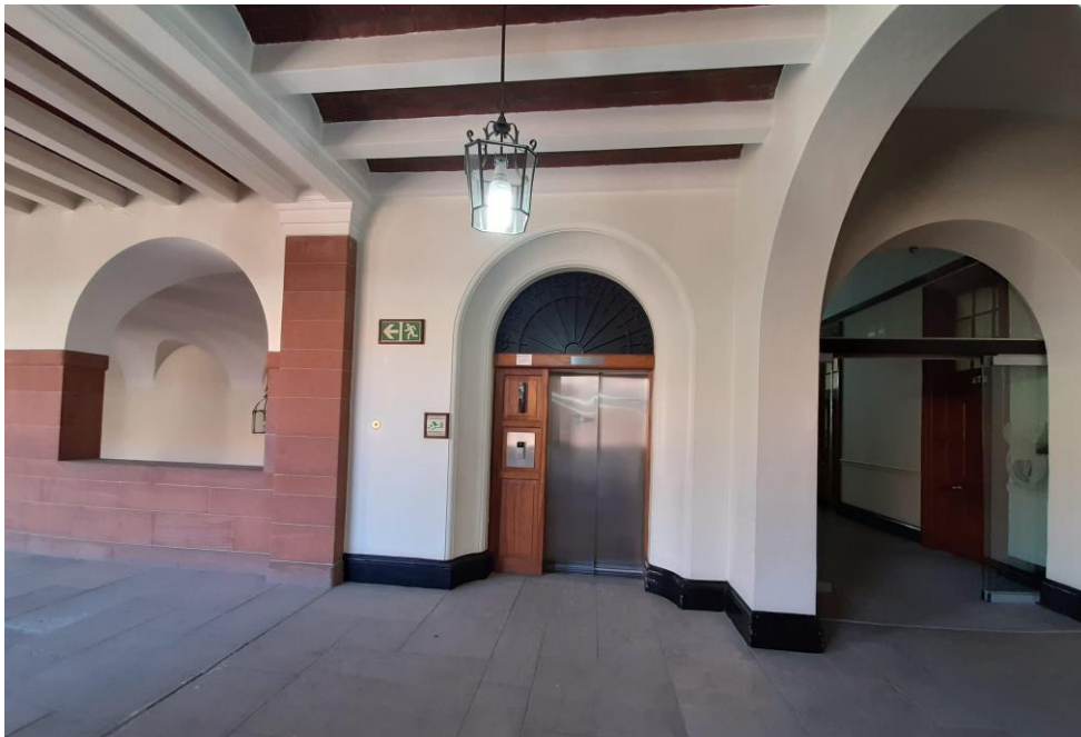
Fig. 70_Passenger lift for the public replaced along the northern side of the main staircase (Source: tsica heritage consultants, 09.07.2019)
