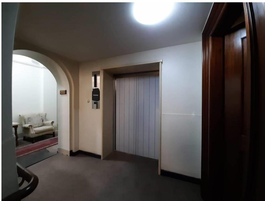
Fig. 59_Goods Delivery Lift replaced on first floor level (Source: tsica heritage consultants, 09.07.2019)
