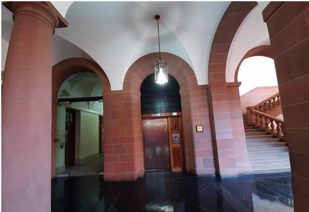
Fig. 53_Passenger lift replaced on first floor level and wooden cladding put back in place without any damage (Source: tsica heritage consultants, 09.07.2019)
