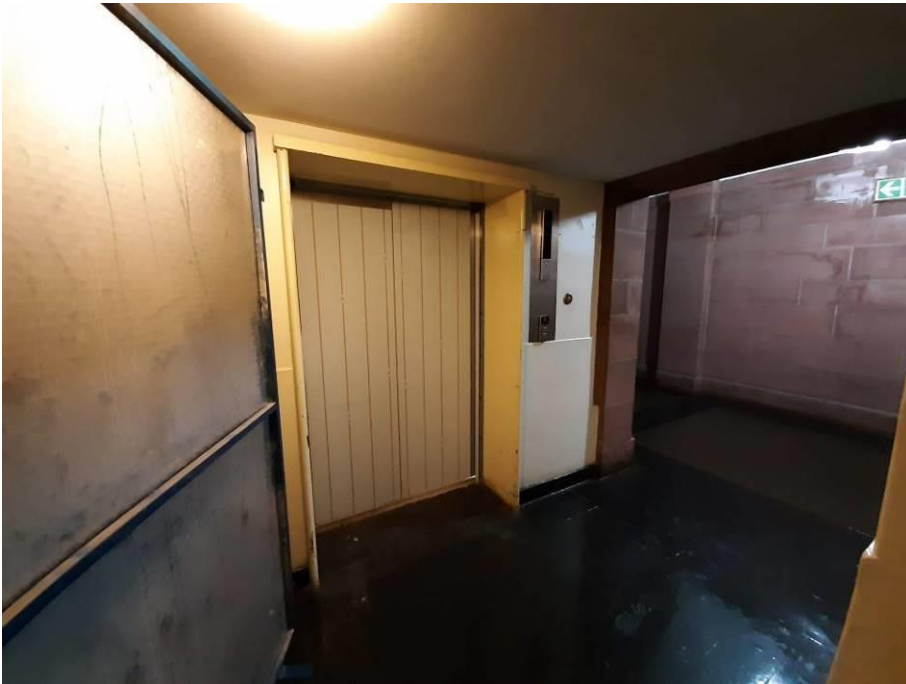
Fig. 75_Goods Delivery Lift replaced on ground floor level (Source: tsica heritage consultants, 09.07.2019)
