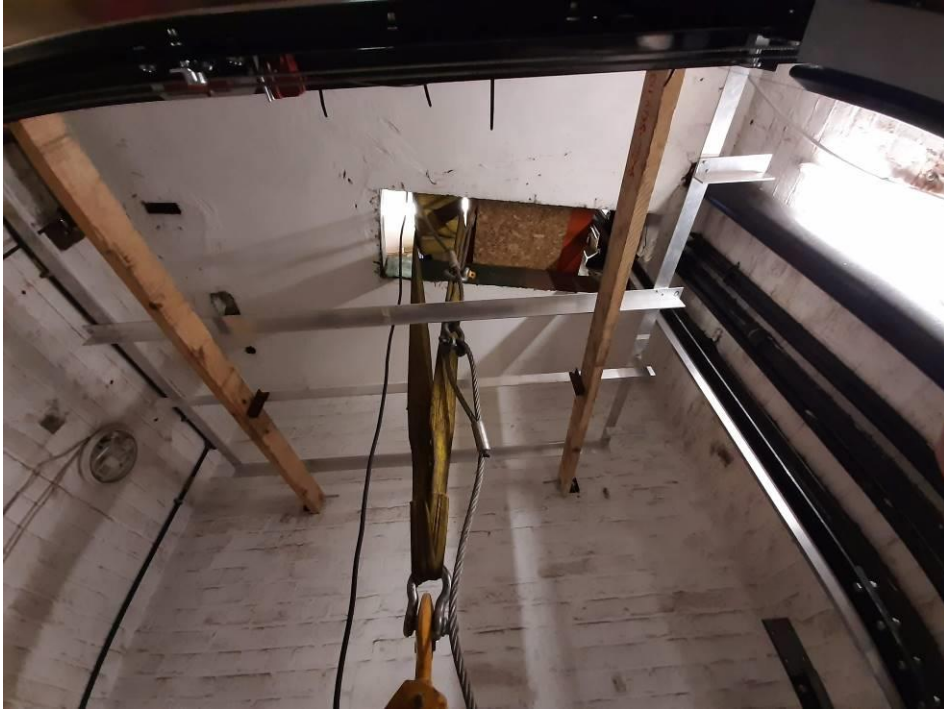
Fig. 84_Lift shaft located in the East wing (Source: tsica heritage consultants, 09.07.2019)
