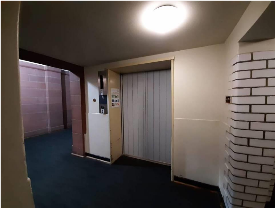
Fig. 58_Goods Delivery Lift replaced on ground floor level (Source: tsica heritage consultants, 09.07.2019)
