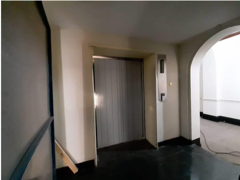
Fig. 77_Goods Delivery Lift replaced on second floor level (Source: tsica heritage consultants, 09.07.2019)
