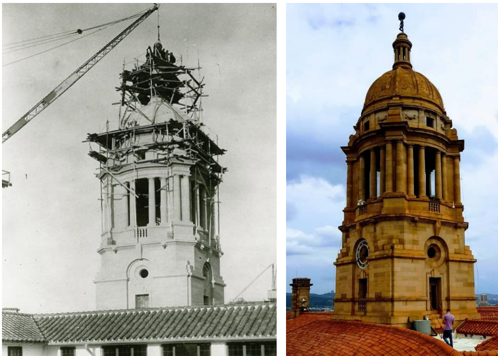
Fig. 12 & 13_Clock Tower during construction in 1912 (left); Clock Tower in 2019 (right) ( http://www.theheritageportal.co.za/article/birth-union-buildings , tsica heritage consultants 2019)
