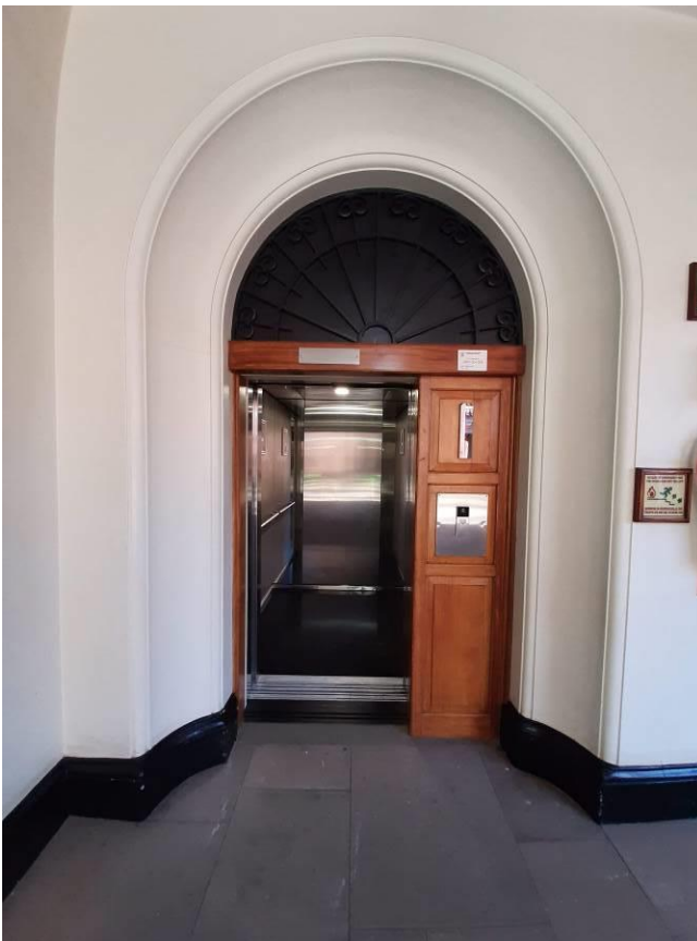
Fig. 74_Passenger lift for the public replaced along the southern side of the main staircase, all wooden cladding was removed and put back without damage (Source: tsica heritage consultants, 09.07.2019)
