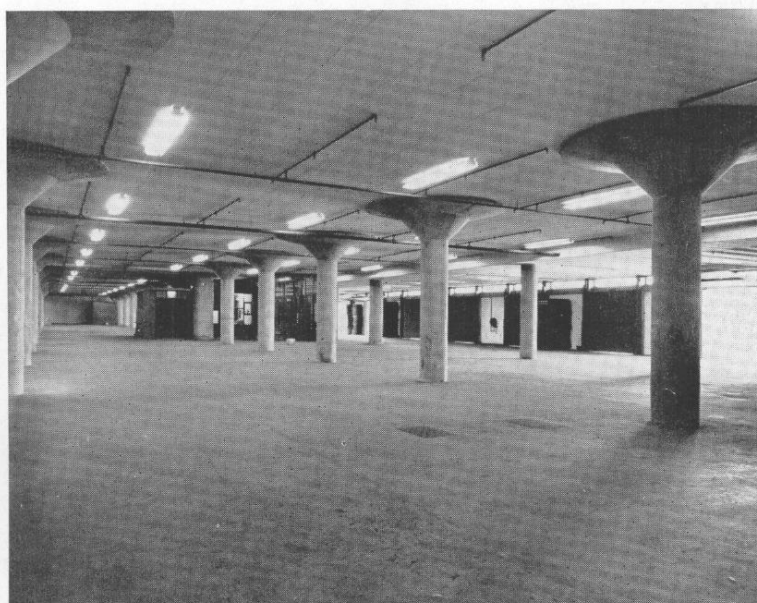
General view of the cargo floor.
