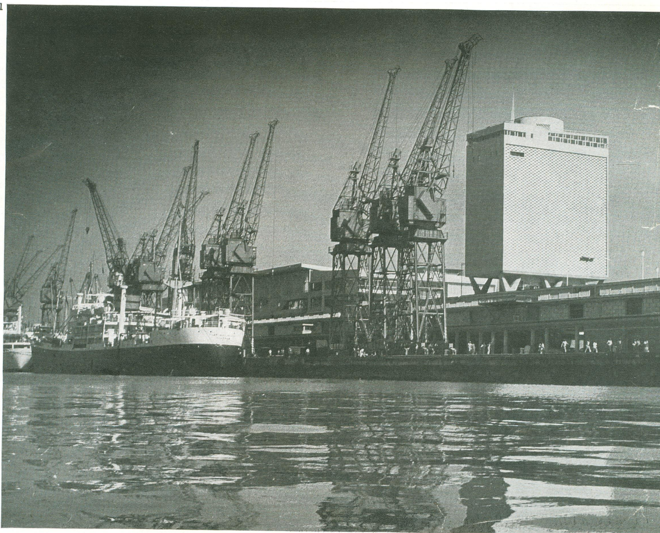
1, looking south-west from the bay, with the 12-storey administration block on the right.
