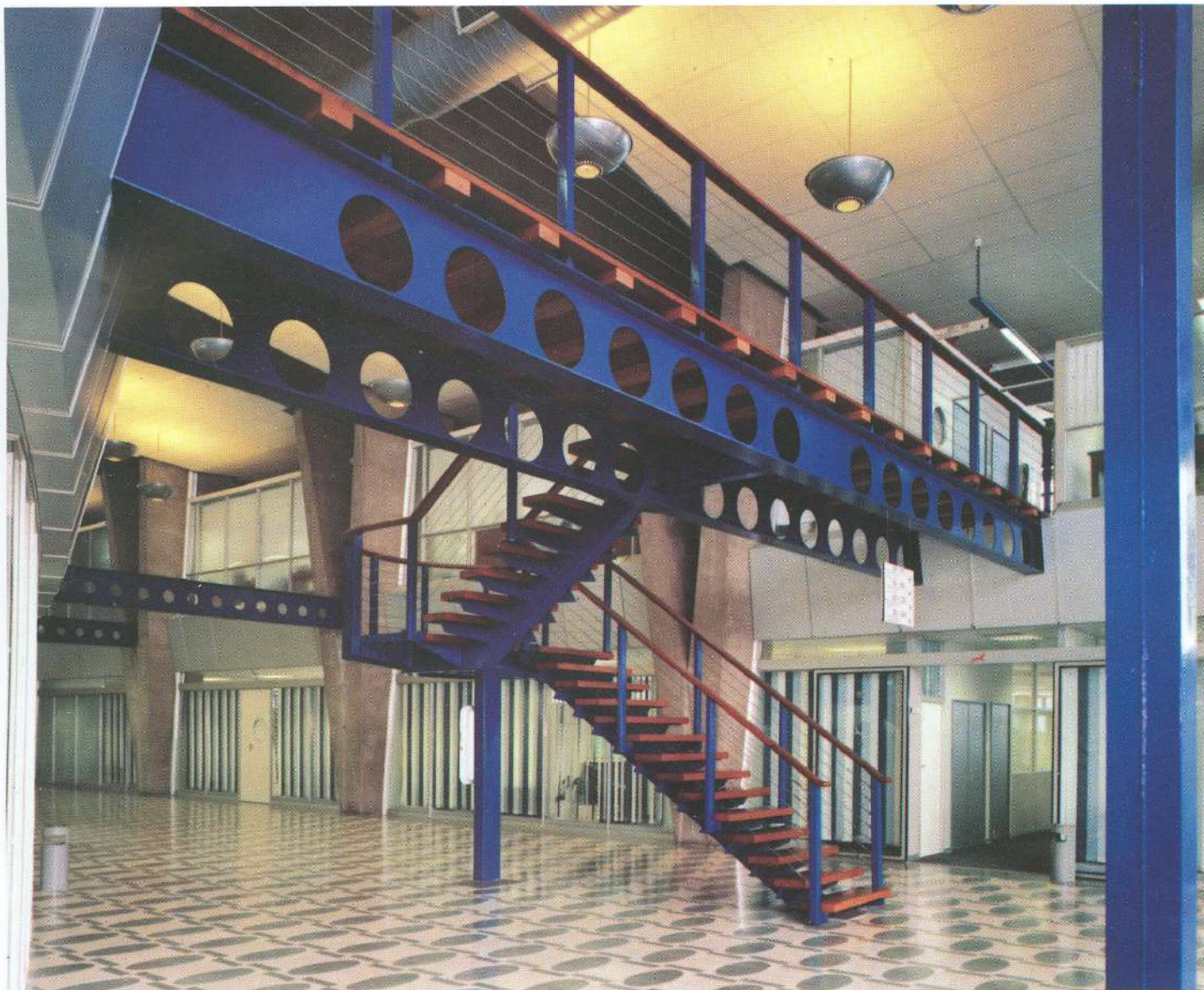
Above: Bridge linking mezzanines over street. Re-used teak planking and handrails.
