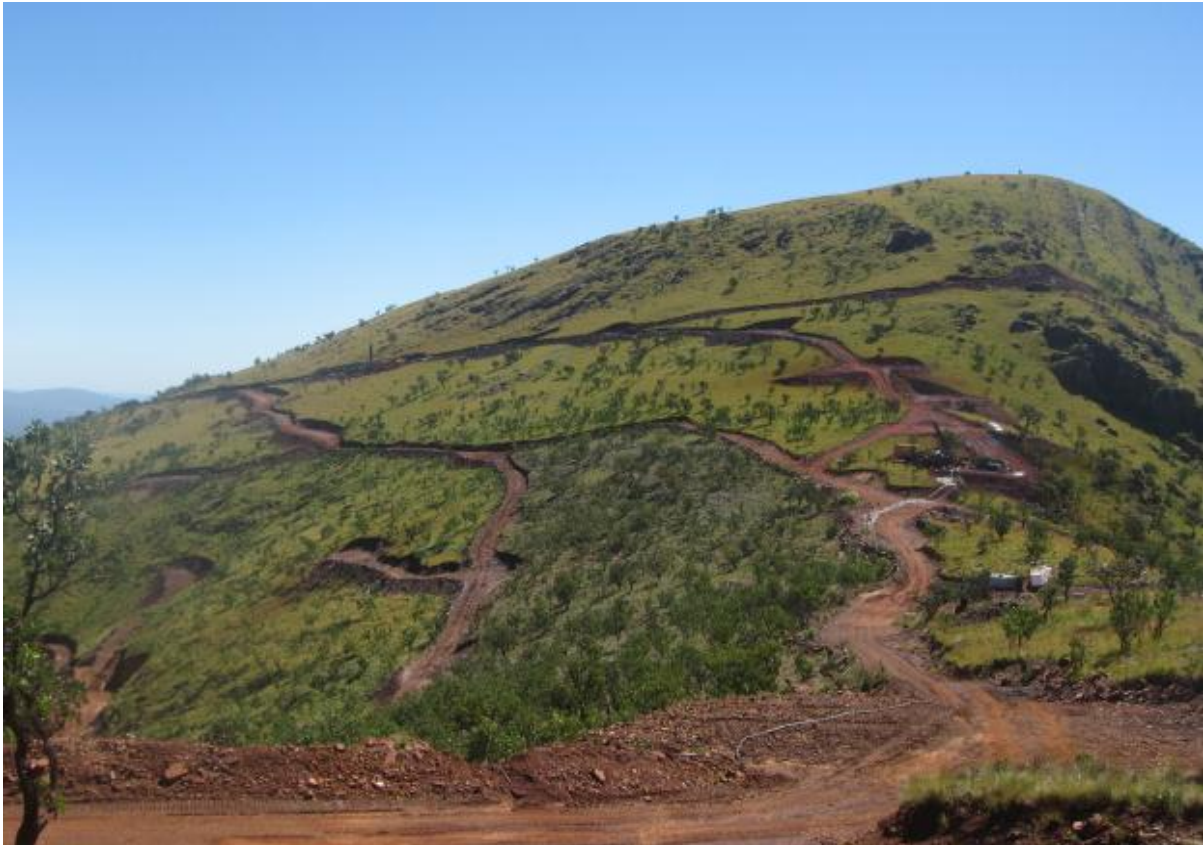
Photo 1: Aerial photograph illustrating the gravel roads on the contravened site
