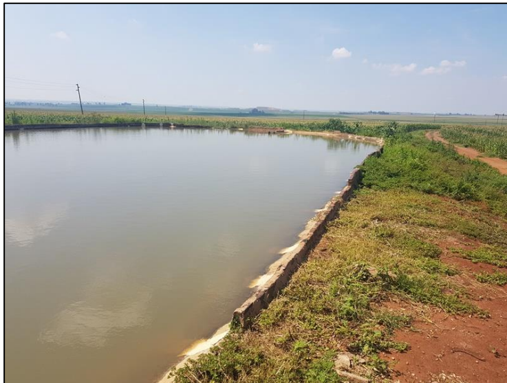
Figure 3-9: A water supply dam in the project area.
