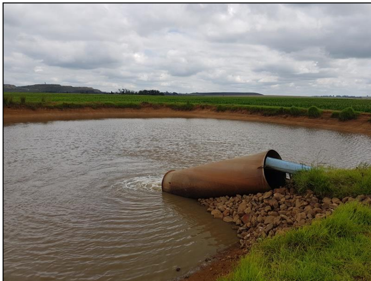
Figure 3-4: A water supply dam in the project area.
