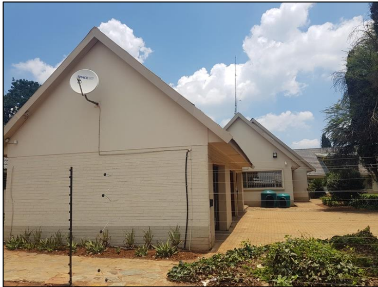
Figure 5-7: View of a Contemporary Period farmhouse residence at Site EXIGO-VGF-CP01.
