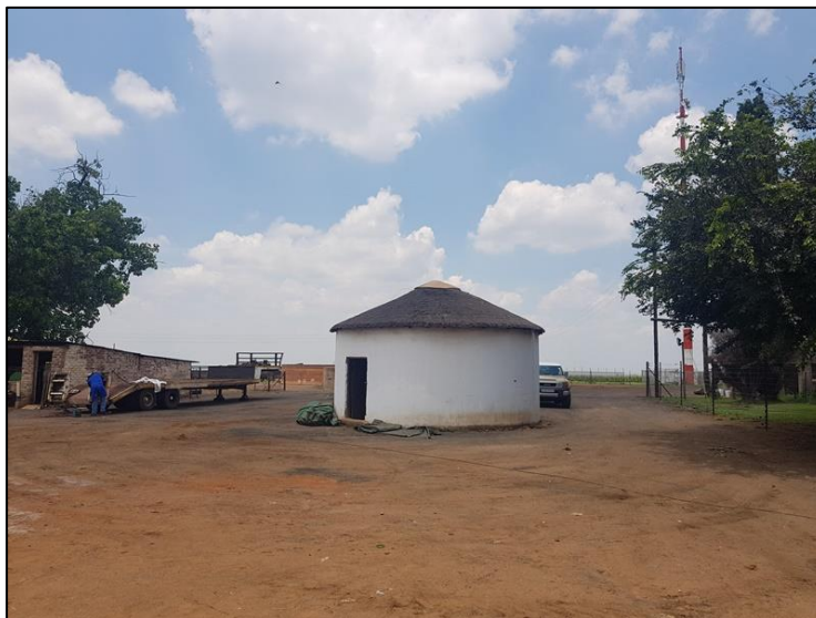
Figure 5-8: View of a Contemporary Period rondavel at Site EXIGO-VGF-CP01.
