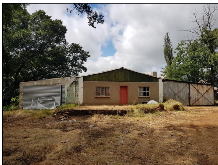
Figure 5-2: View of a building at Site EXIGO-VGF-HP01.
