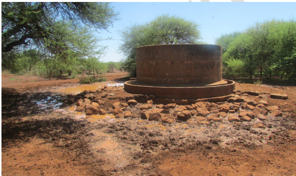
Figure 72: An overview of the structure noted on the area proposed for blasting.
