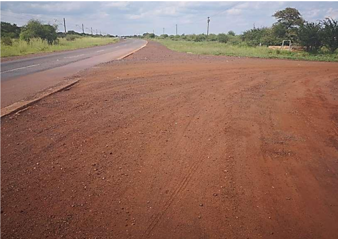
Figure 13: R510 Intersection with gravel road A
