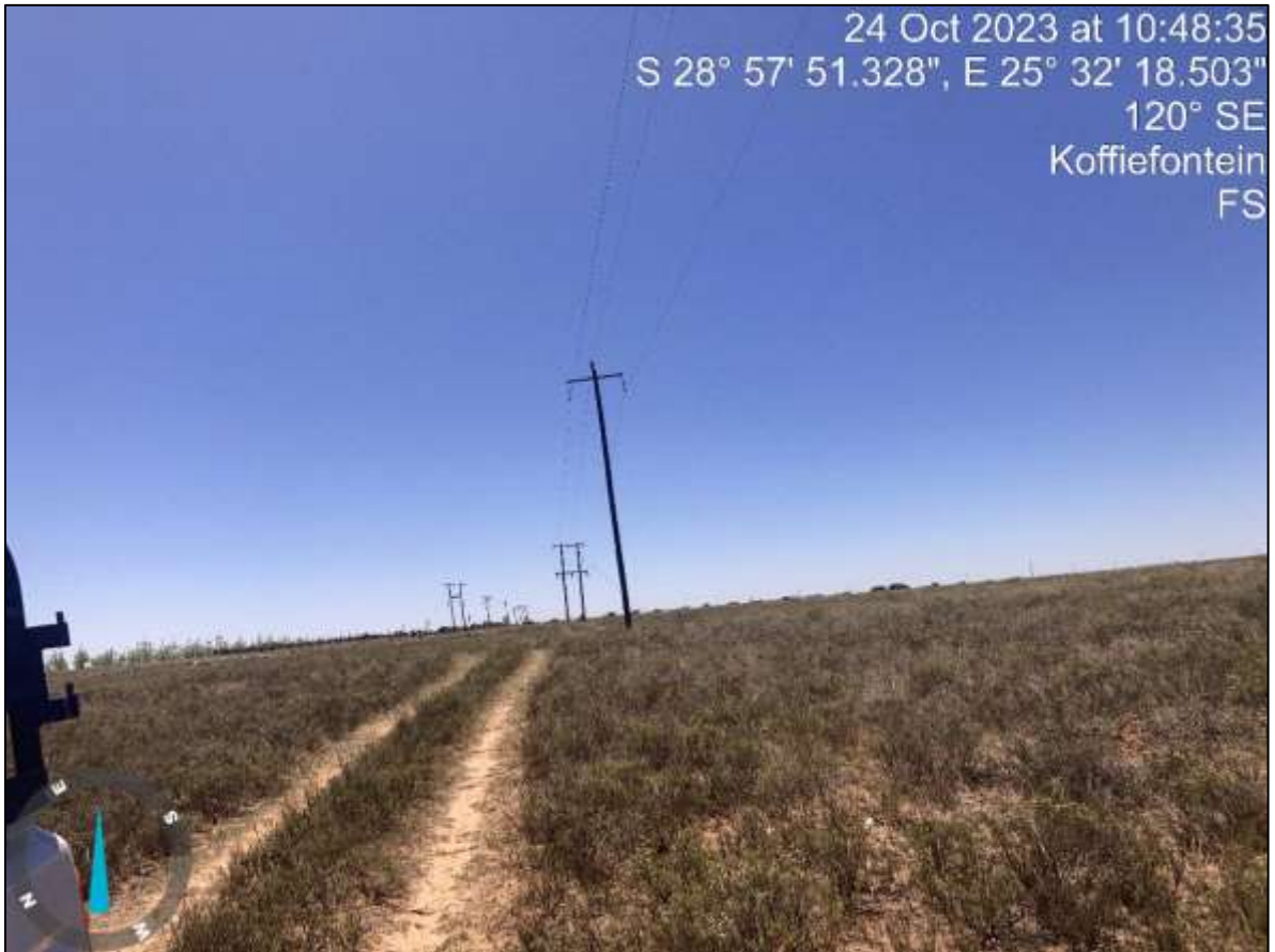
Figure 8: Powerlines running through the prospecting area.
