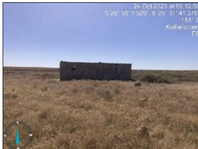
Figure 43: A ruin farm worker house.
