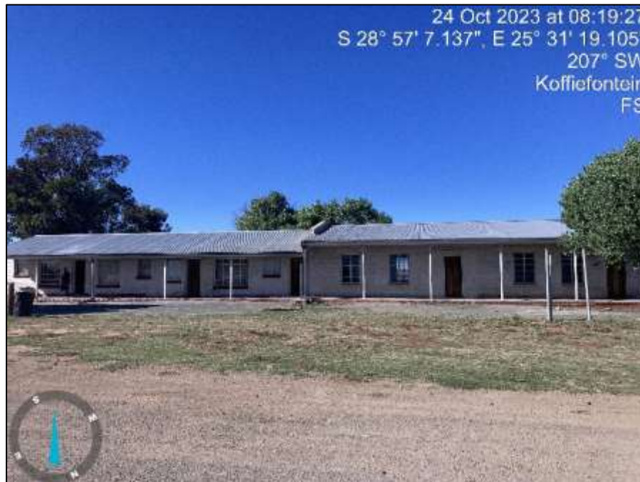
Figure 34: The old Lawrence Primary School building.
