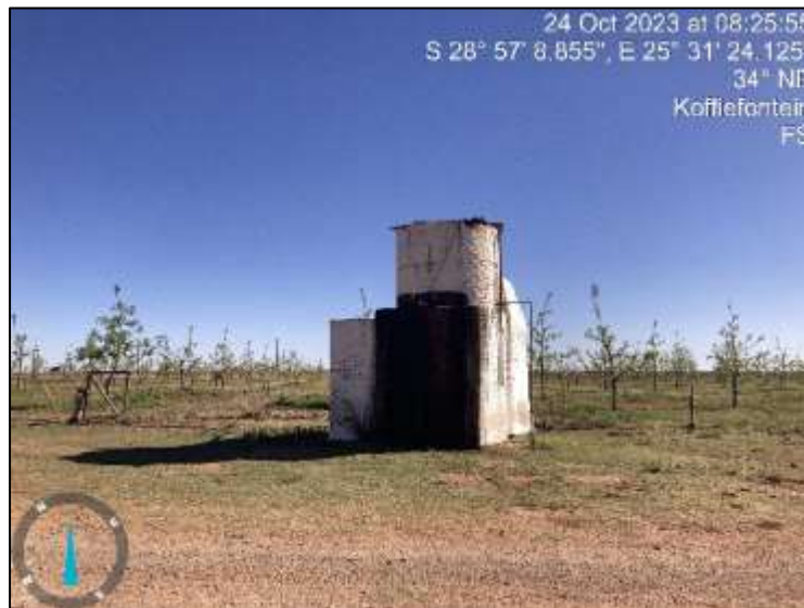
Figure 52: A pump that was previously used as a shower located outside of the prospecting area.
