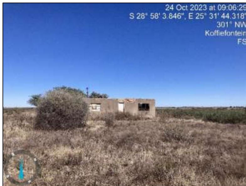
Figure 47: A ruin farm worker house.
