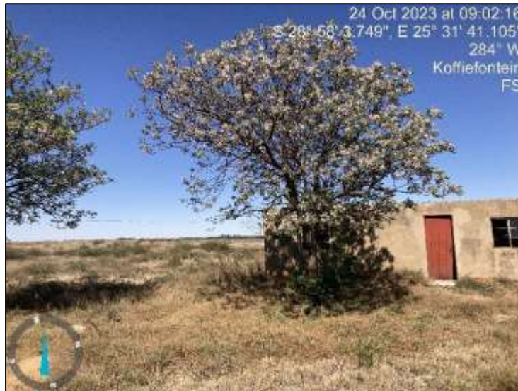
Figure 51: A ruin farm worker house.
