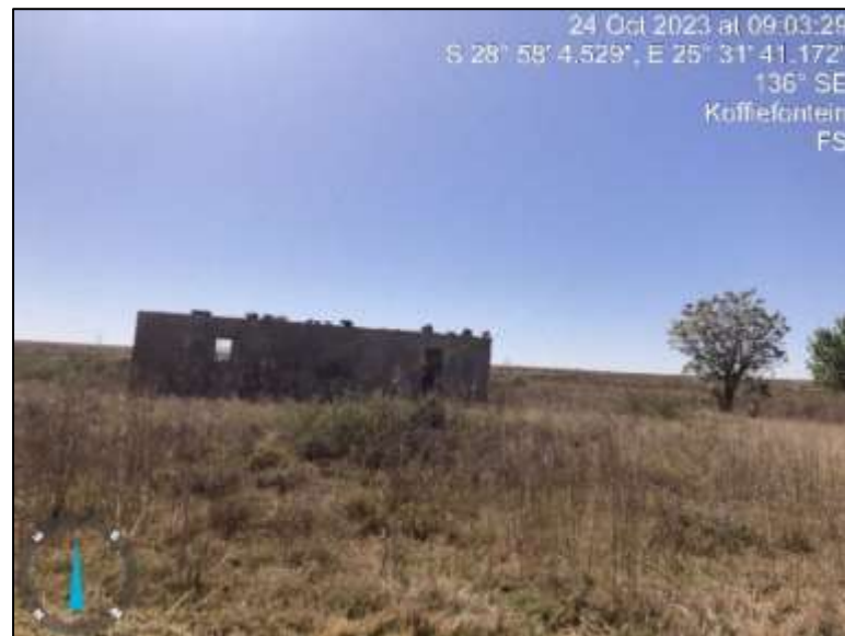
Figure 45: A ruin farm worker house.
