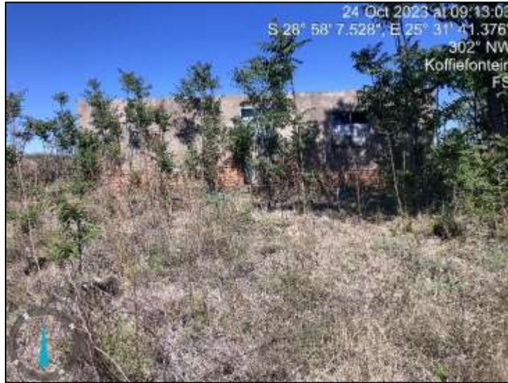
Figure 50: A ruin farm worker house.
