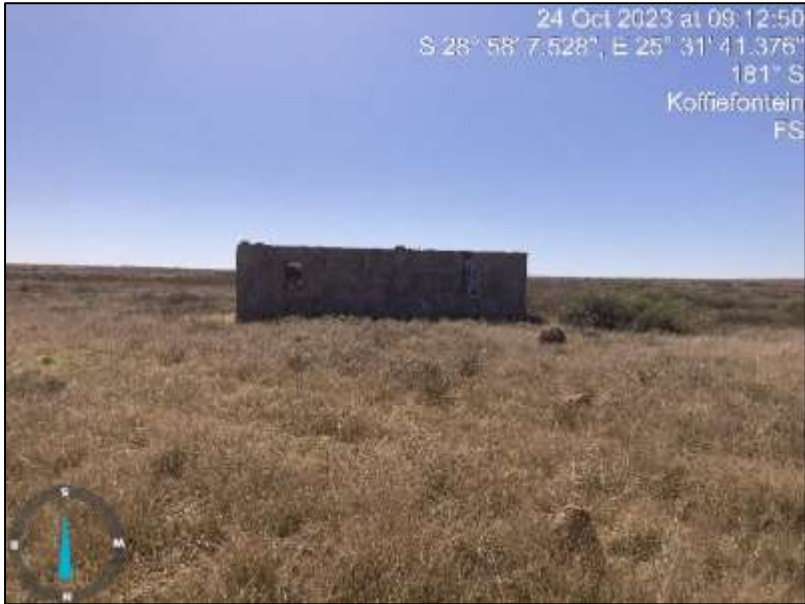
Figure 49: A ruin farm worker house.
