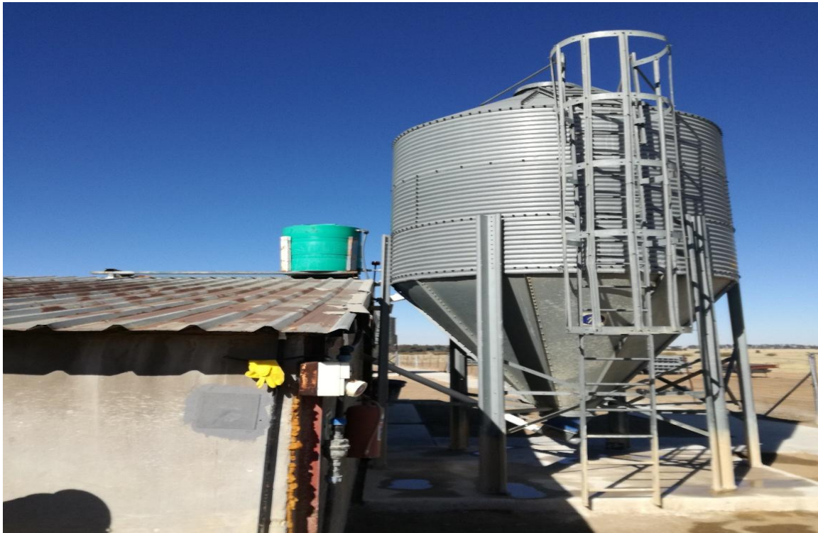
Figure 5 - Feeding silo and green water tank.
