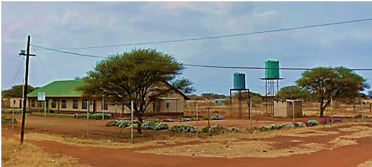
Figure 8-7: Jojo tanks as well as pit latrine at Mononono Clinic
