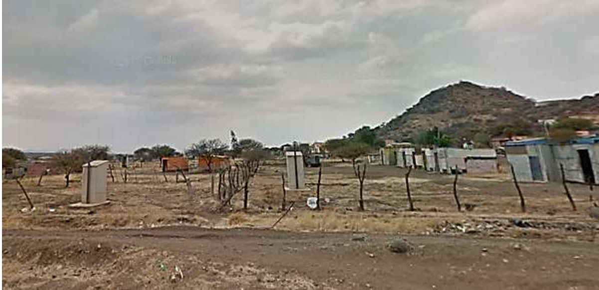
Figure 8-5: VIP toilets in Sefikile
