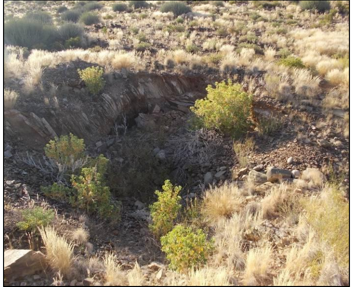
Figure 13: A second excavation into harder bedrock.
