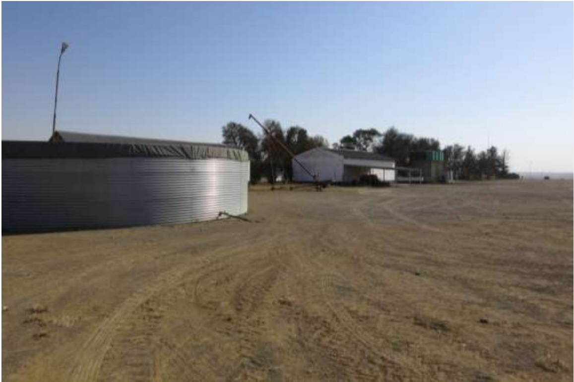
Figure 5: Photograph of a water reservoir, store room and JoJo tanks in the distance (at the existing broiler facility).
