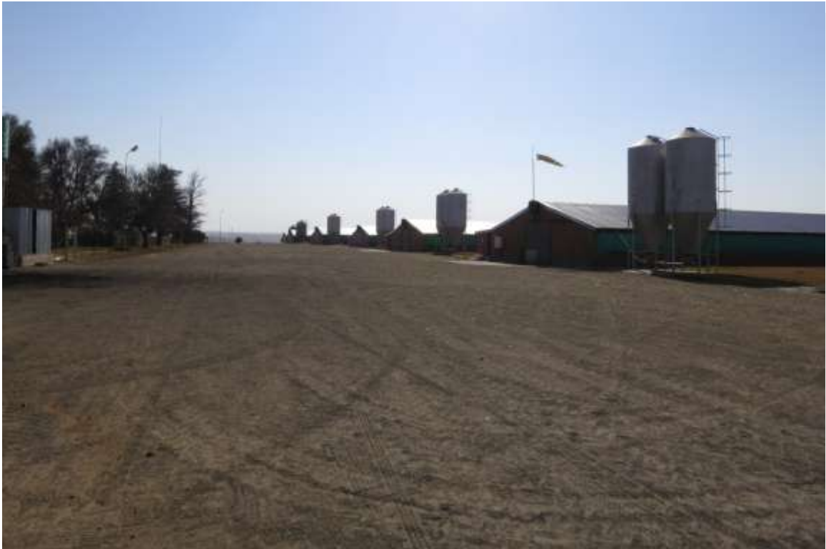
Figure 3: Photograph of the current broiler houses.
