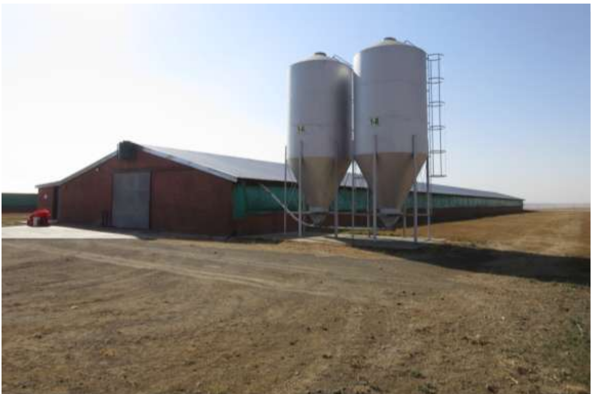
Figure 4: Photograph of an existing poultry house and its feeding silos.
